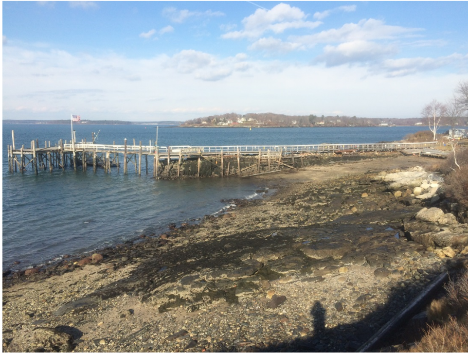
Figure 3: View Looking North
