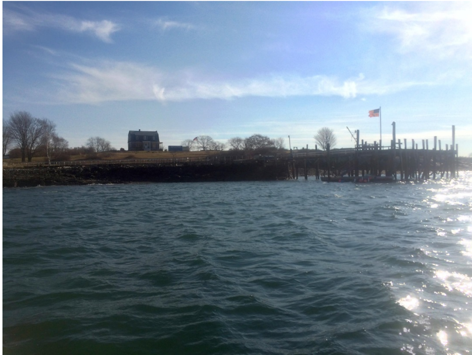
Figure 1: View Looking South
