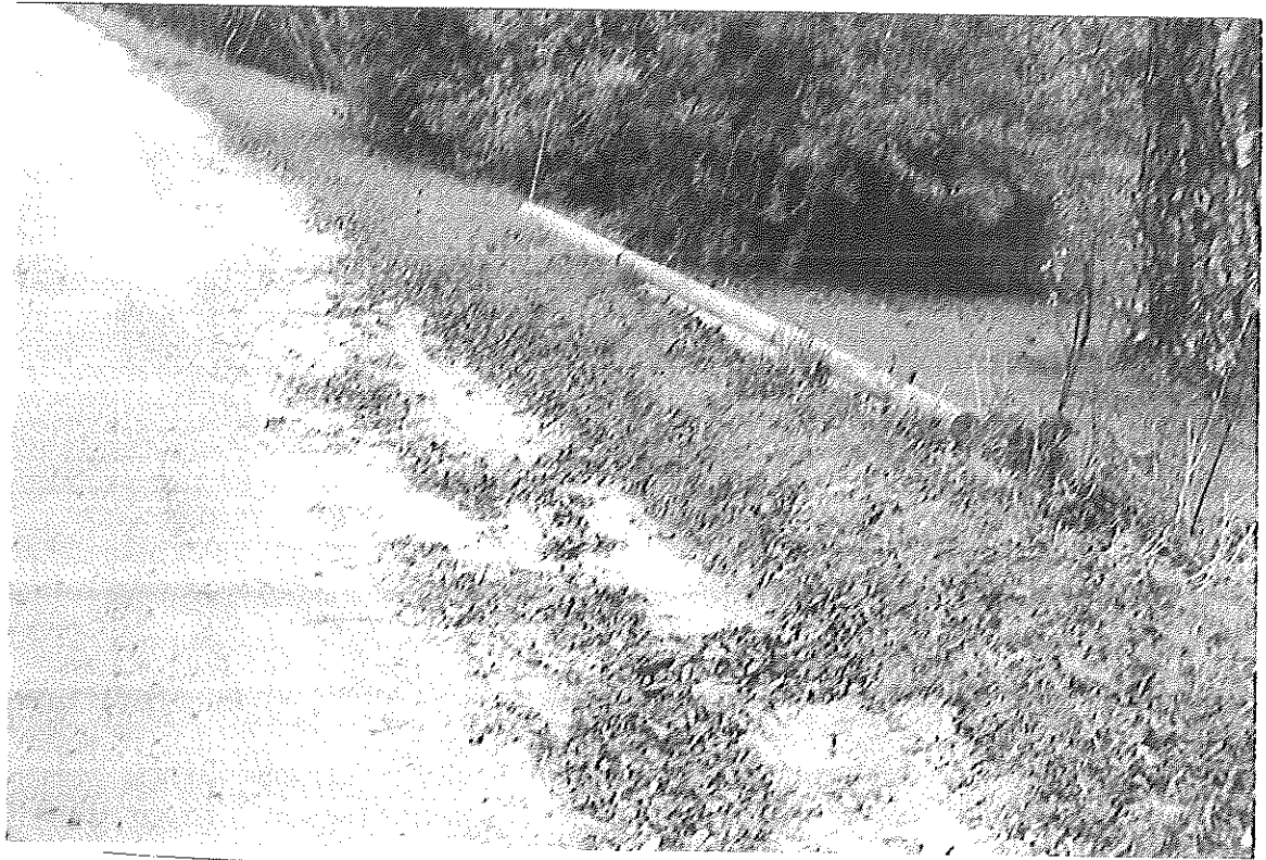
Boards placed here to protect pipe from traffic
