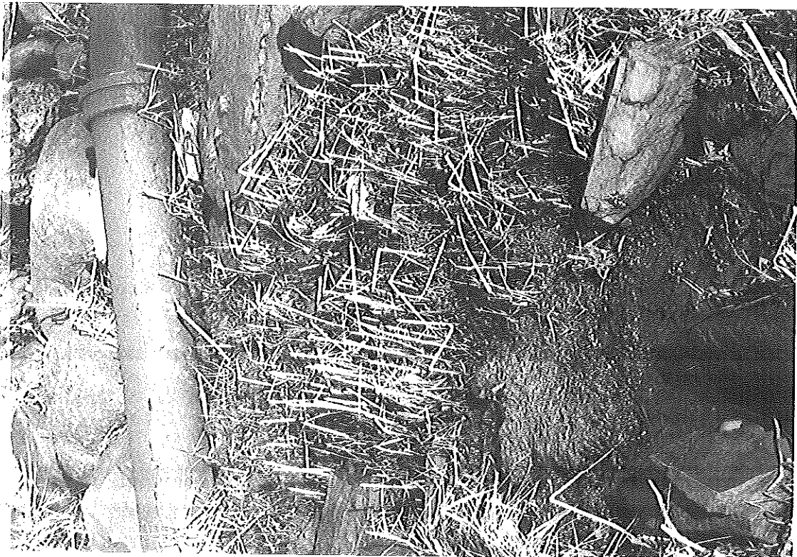
green areas growing by sludge
