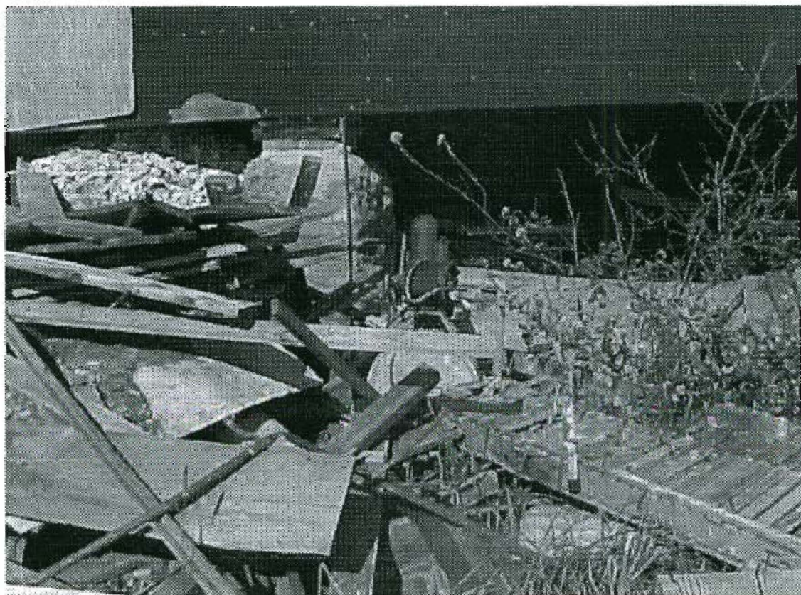
Photo 10: View of remains of existing water pipe.
