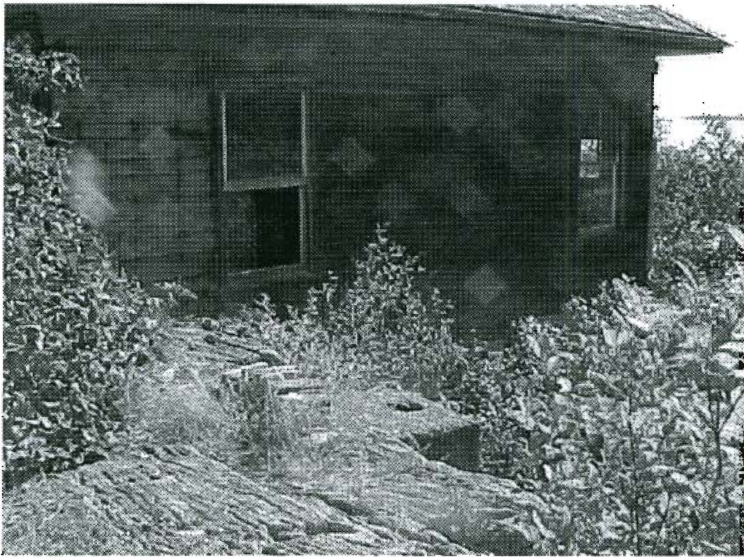
Photo 7: View of north side yard with bedrock in foreground.
