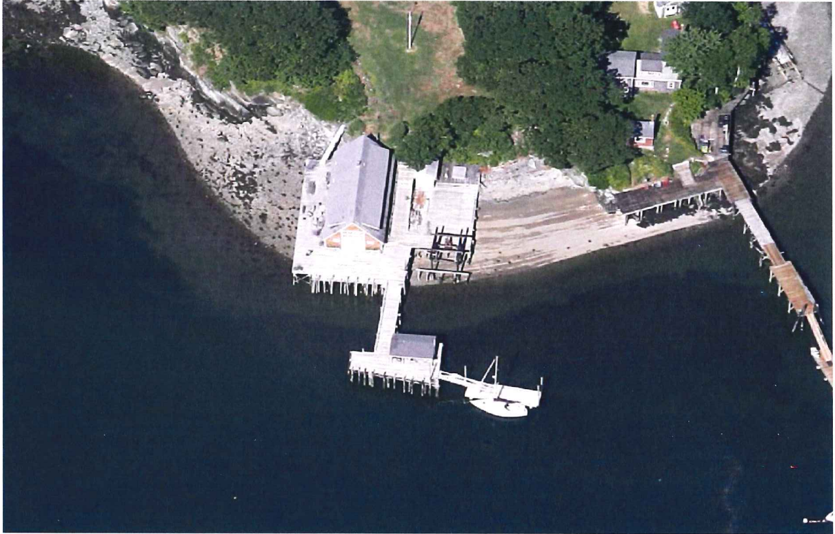
Aerial view of existing pier looking southwest
