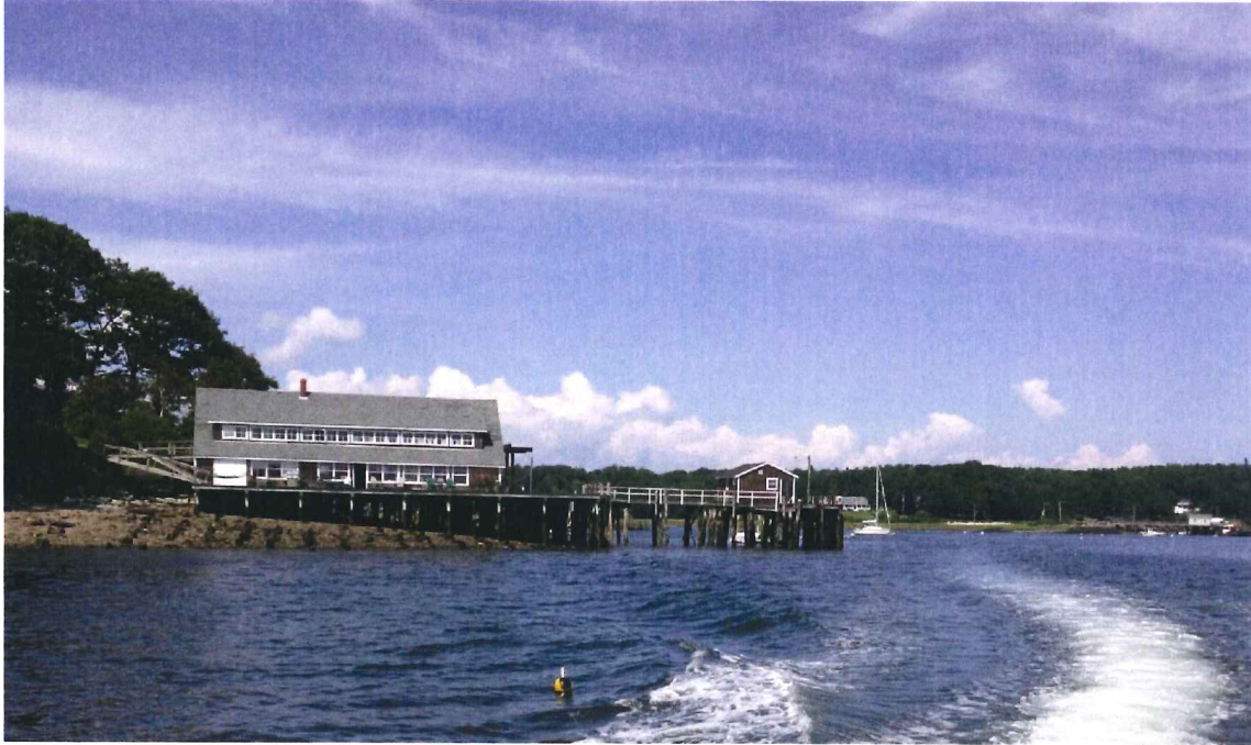
View of existing pier looking north, taken 8-13-2012
