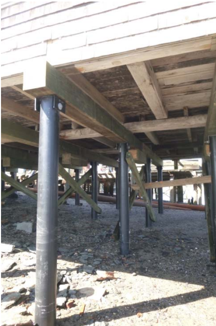
Figure 3. New composite building support piles and heavy timber caps
