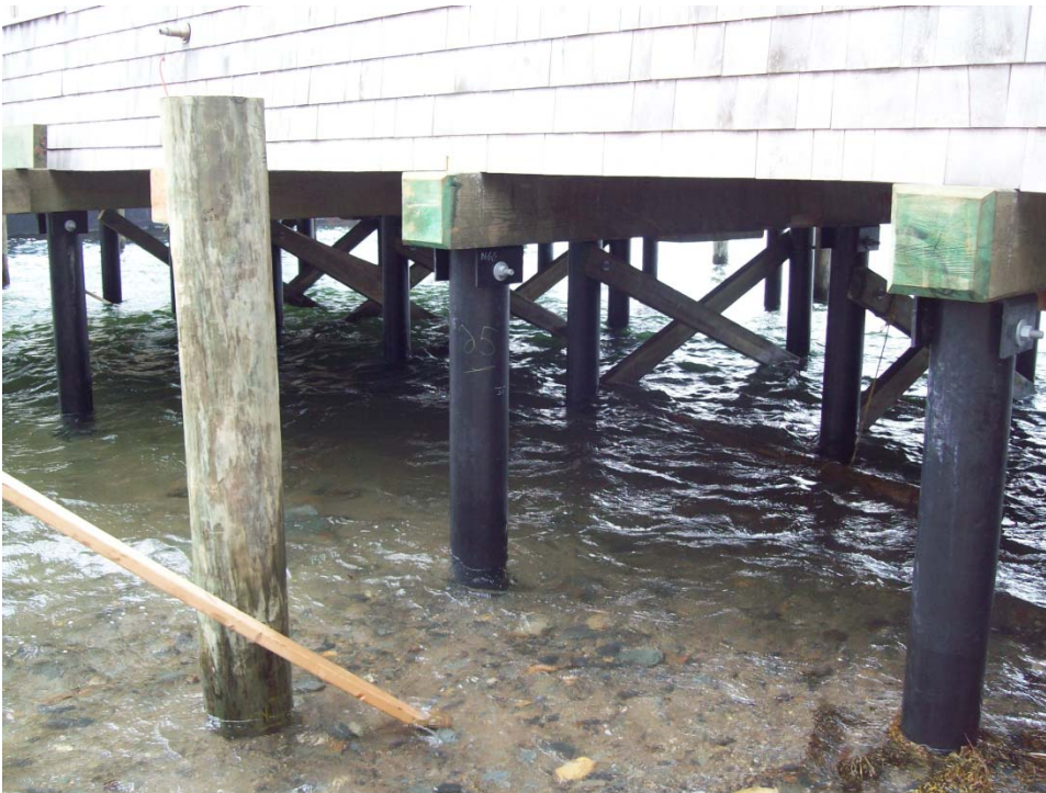
Figure 2. New composite building support piles and heavy timber caps
