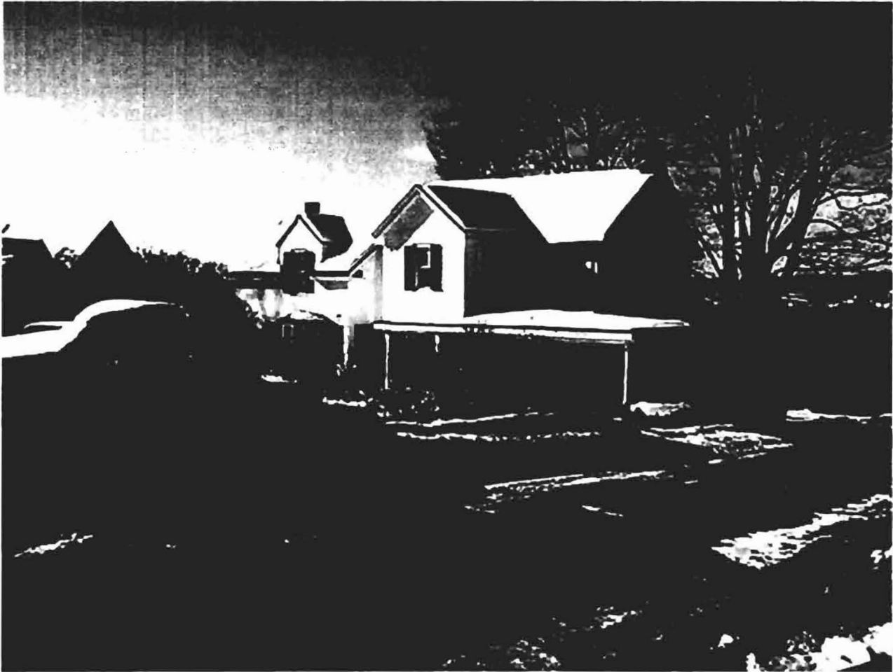
PHOTO OF EXISTING HOUSE FROM THE NORTHEAST.
