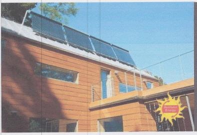
At left is a 120-tube solar hot water collector array installed by ReVision Energy on a passive solar house in Belfast, ME. The system is used to provide domestic hot water and radiant space heating.
