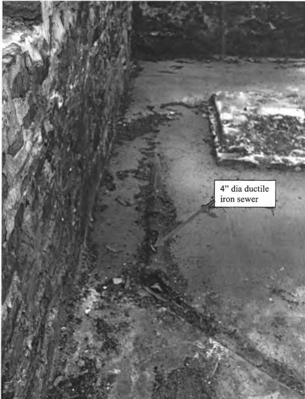
Photo 1: Existing building sewer line
