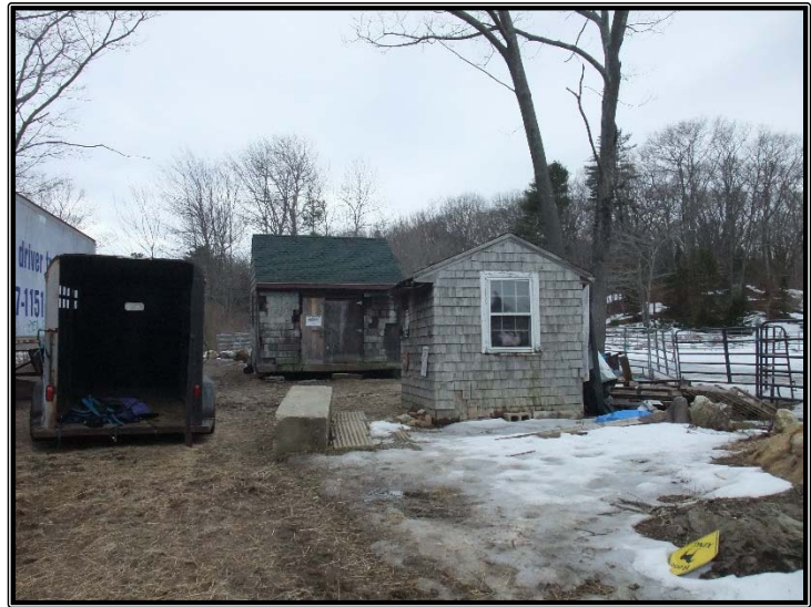
Shed #2 (front) – 8' by 8' Shed #1 is visible in rear
