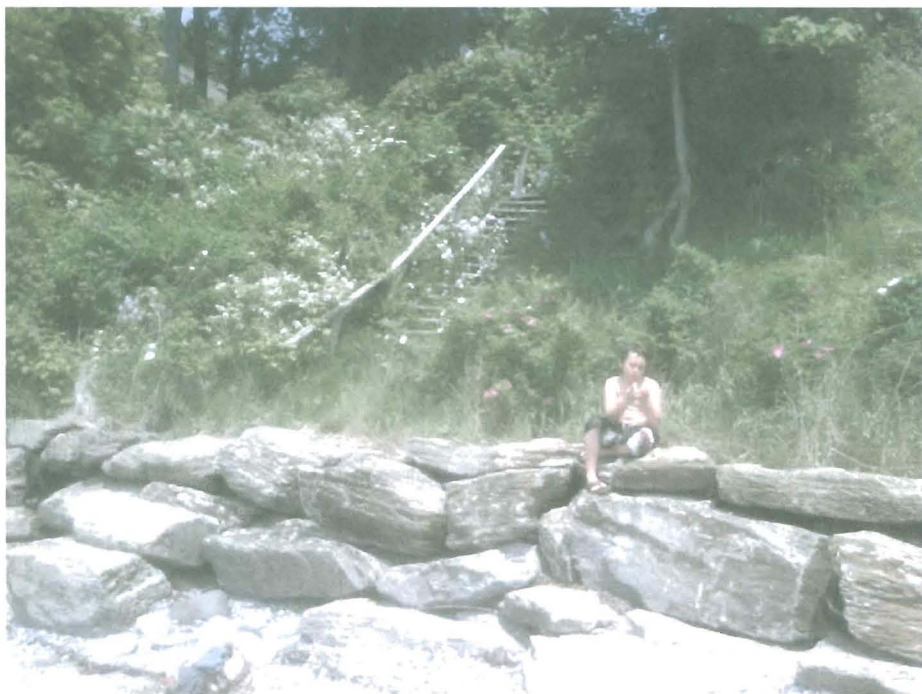
Summertime View showing vegetated slope
