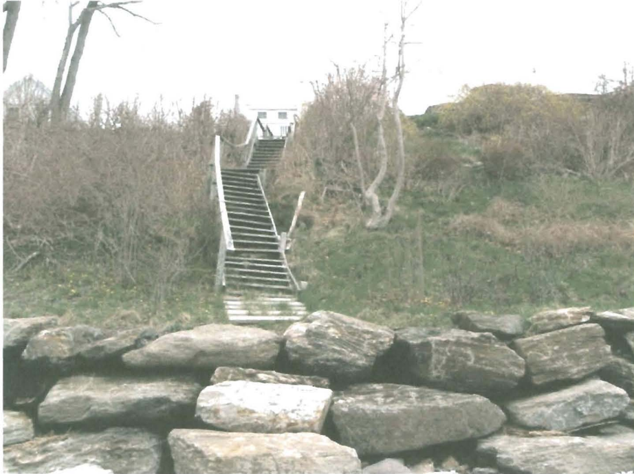
View of Existing Stair from Beach. New stair follows existing alignment
