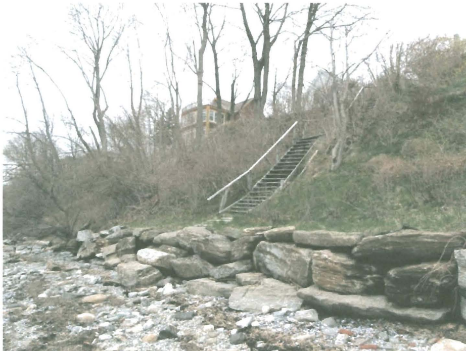
Oblique View of Stair from Beach
