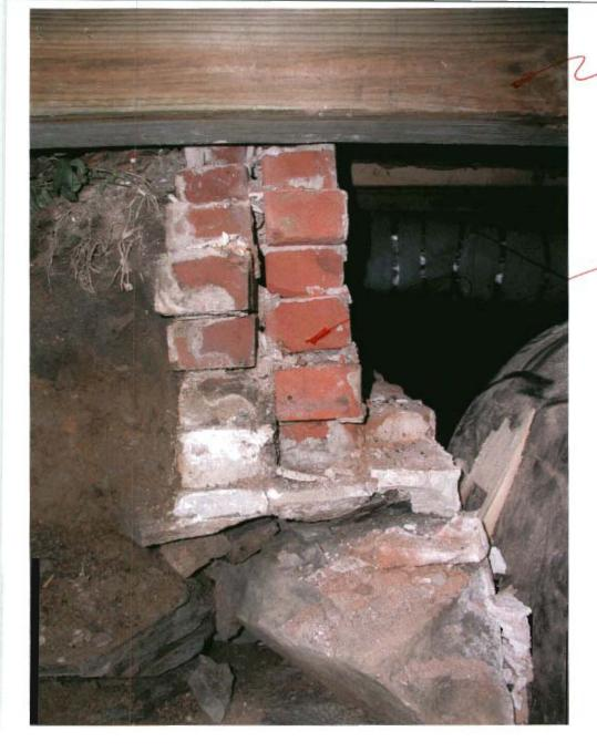
EXISTING BRICK-FOUNDATION TO BE REPAIRED AND PARTIALLY REBUILT.
