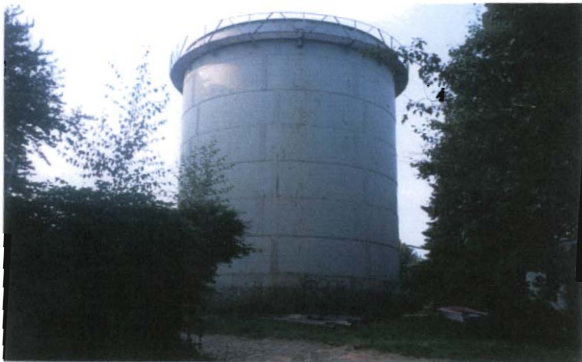
"A" Street Side Looking Southerly
