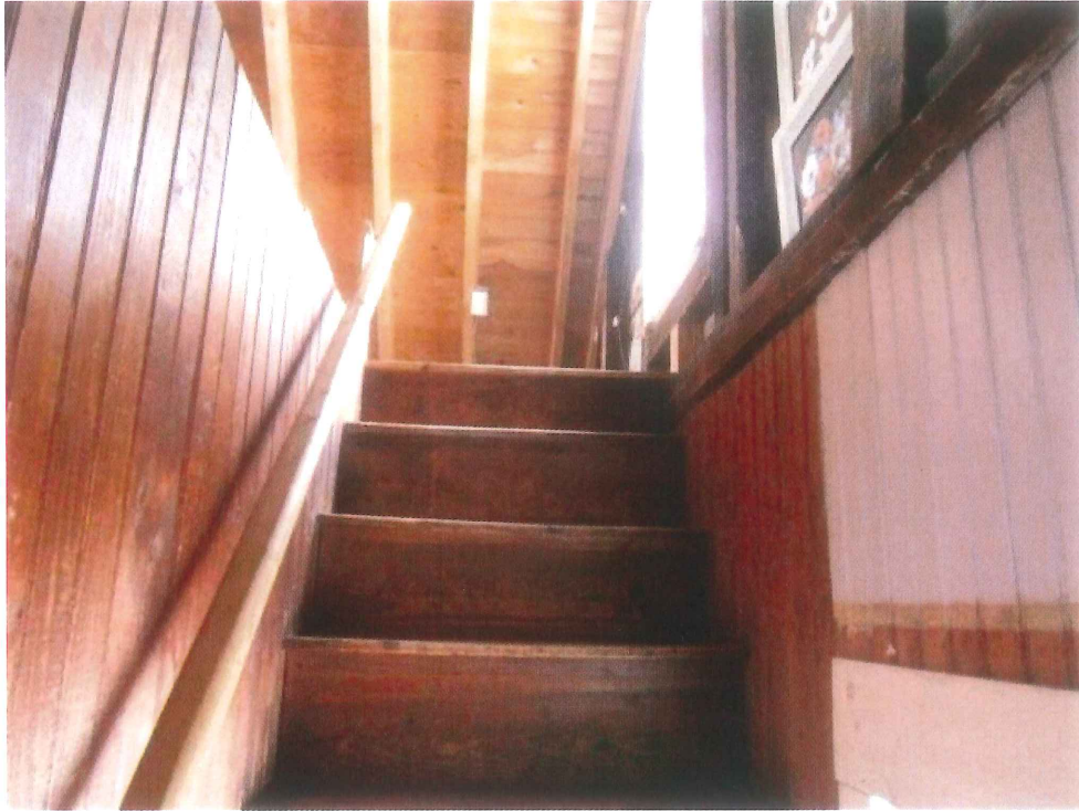
2 nd Floor – Stairs to Attic
