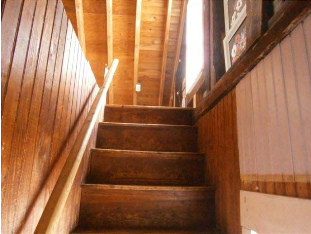
2 nd Floor – Stairs to Attic
