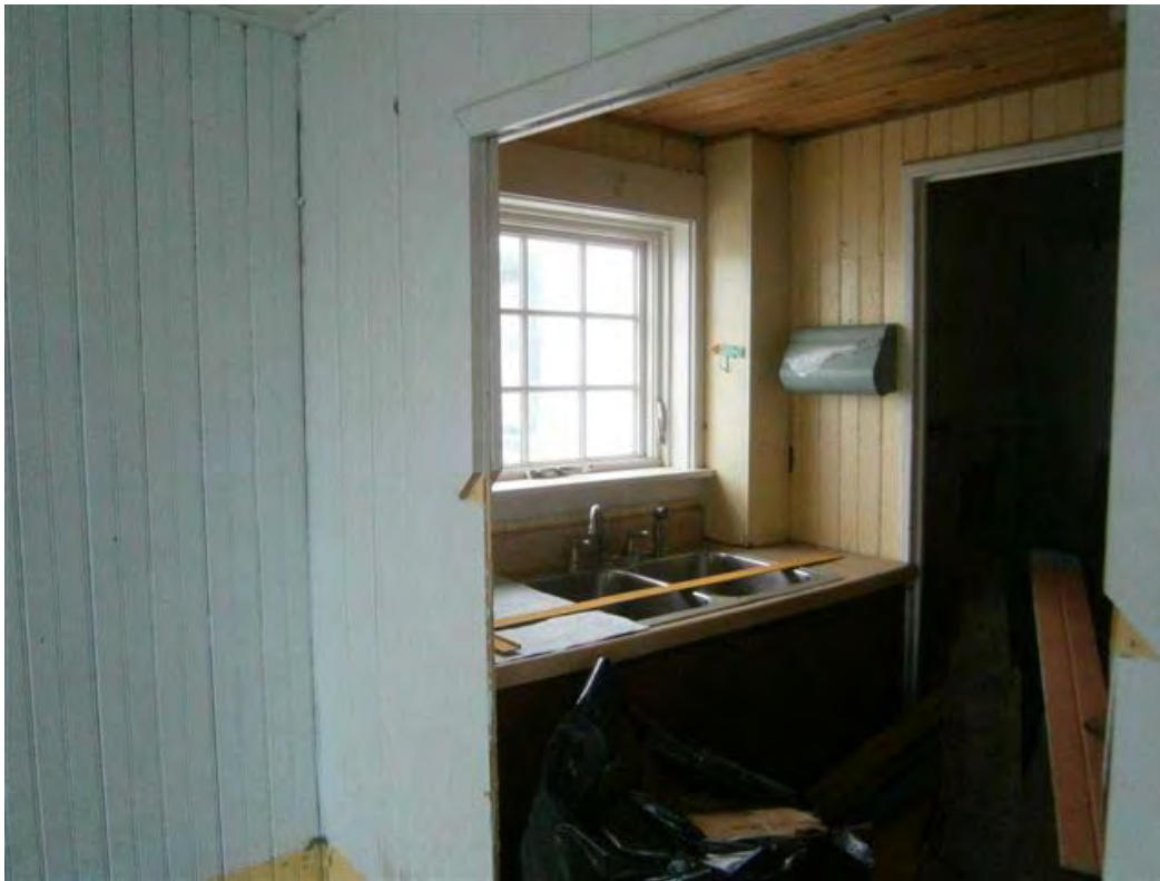
1 st Floor - Kitchen
