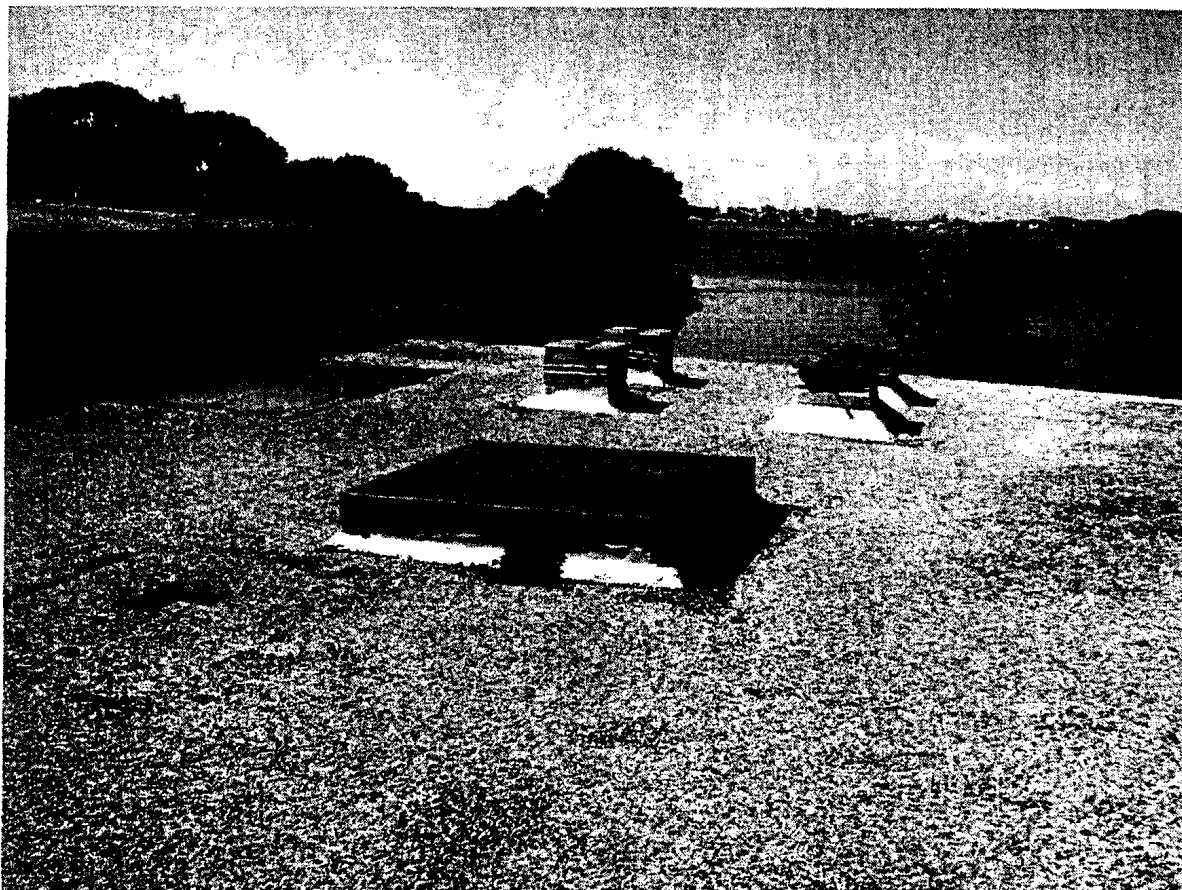
Peaks Island Building. Lower roof to be reroofed. All penetrations to be removed.
