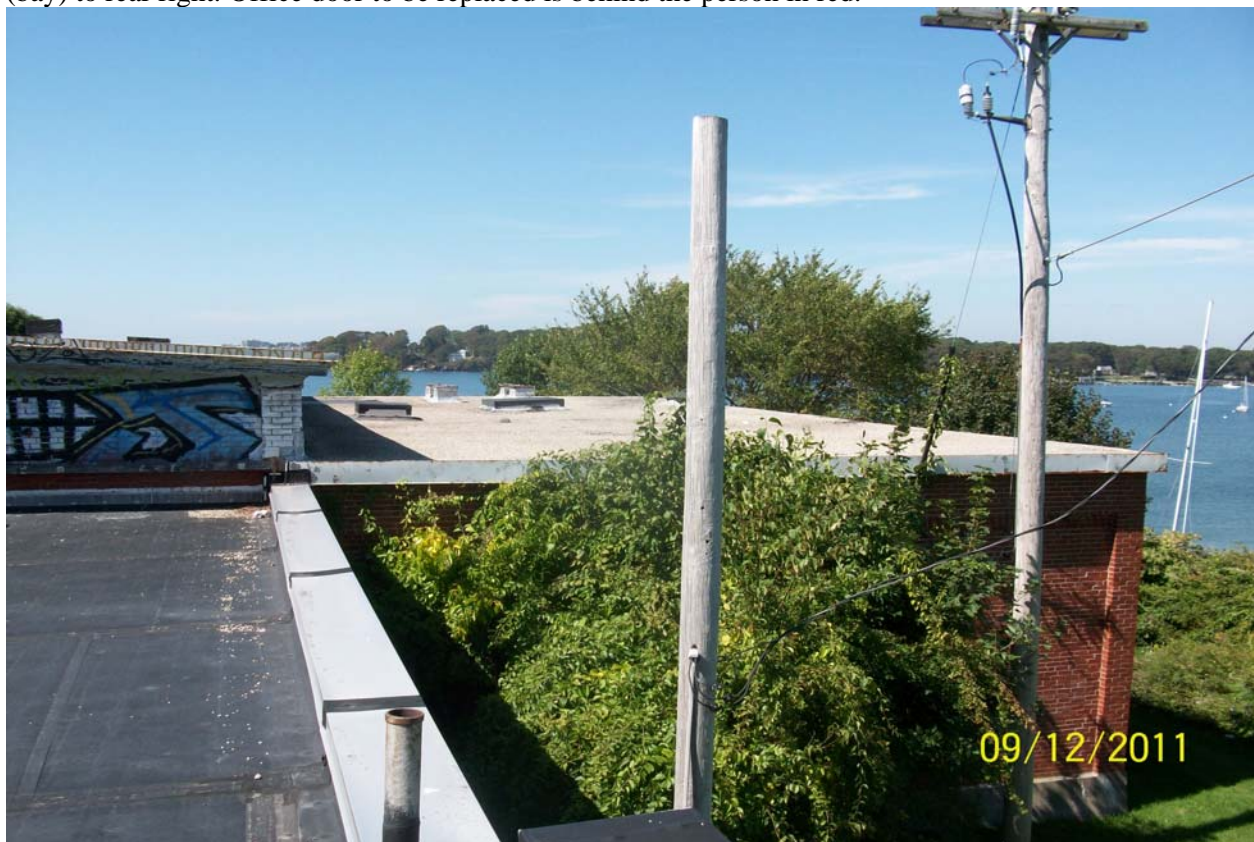
Peaks Island: Lower roof to be reroofed to the right.
