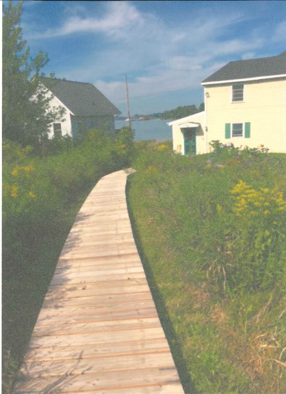
view of walkway
