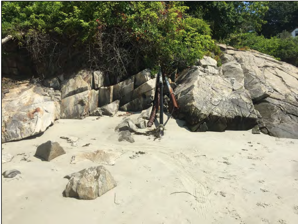
Photo 3. Peaks Island facing northeast. Cable will be armored where it runs over ledge and anchored in place with U bolts.
