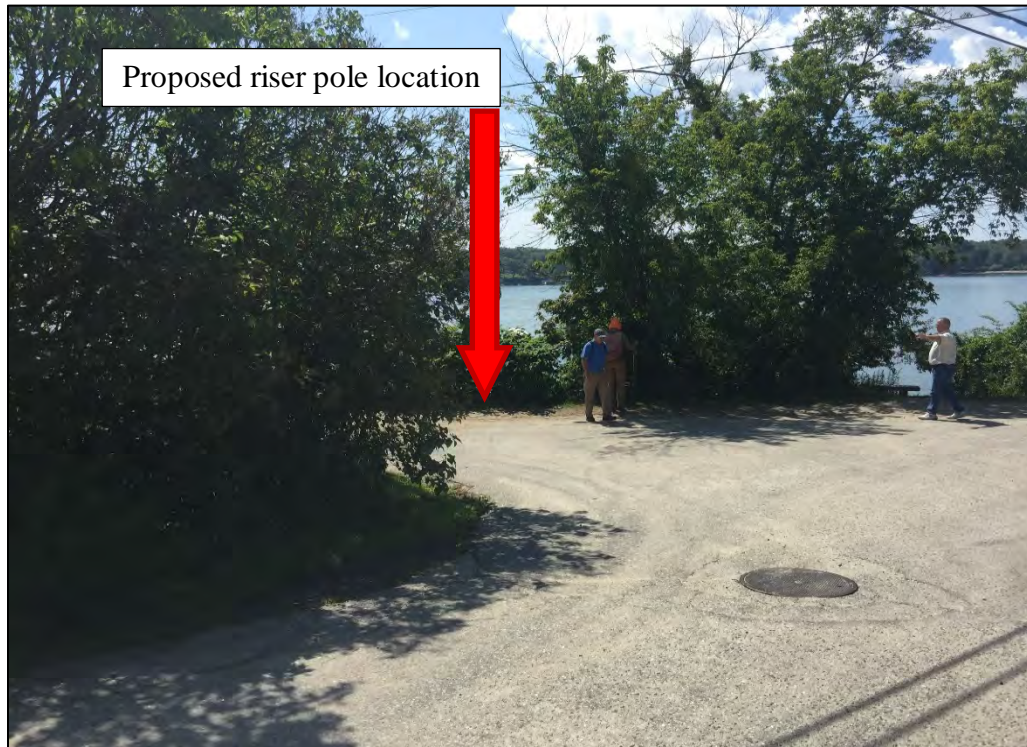
Photo 1. Peaks Island. Facing south from Greenwood Street to location of new riser pole. One tree <3" DBH may be removed or partially limbed at contractors discretion. The cable will be buried passing the bench towards and onto the beach.
