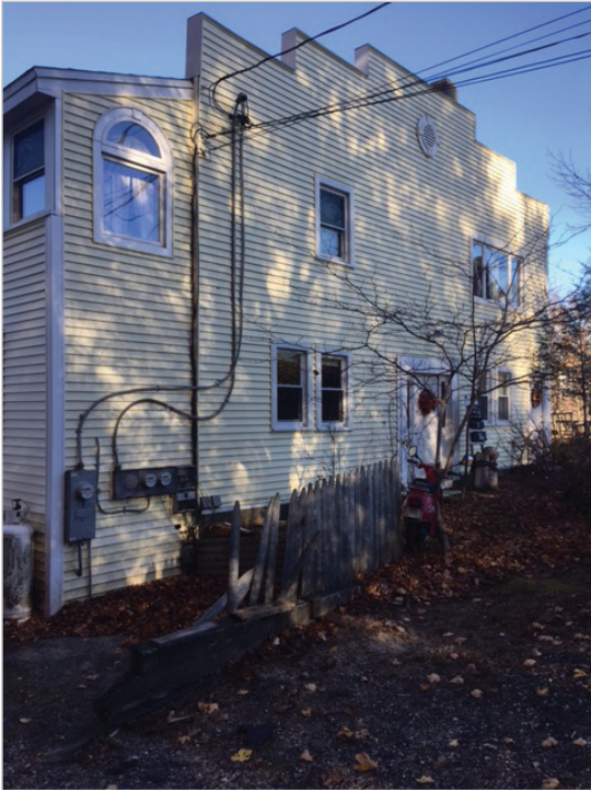
Front (street side)
