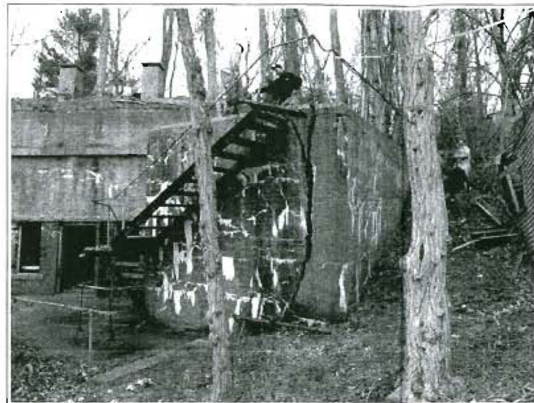
EXTERIOR - EXISTING STAIR ASSEMBLY
