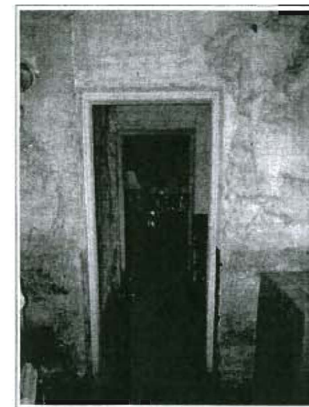
INTERIOR - HALL TO ENGINE ROOM
