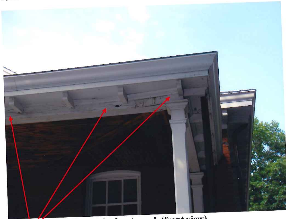
Right front porch (front view)
