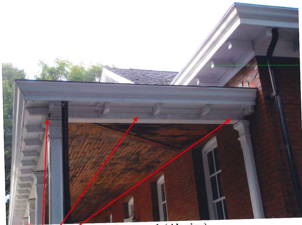
Right front porch (side view)
