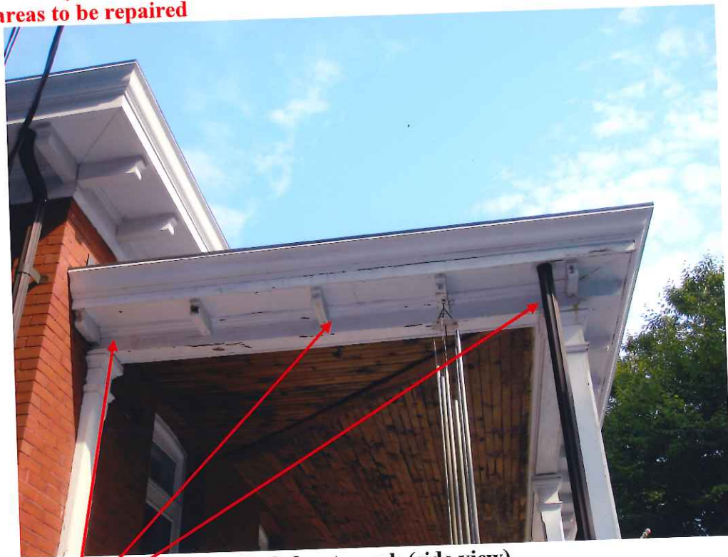
Left front porch (side view)
