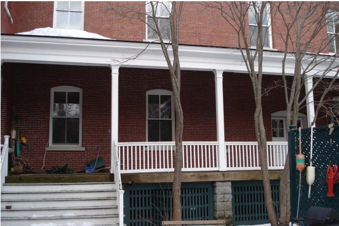
General view of back door.
