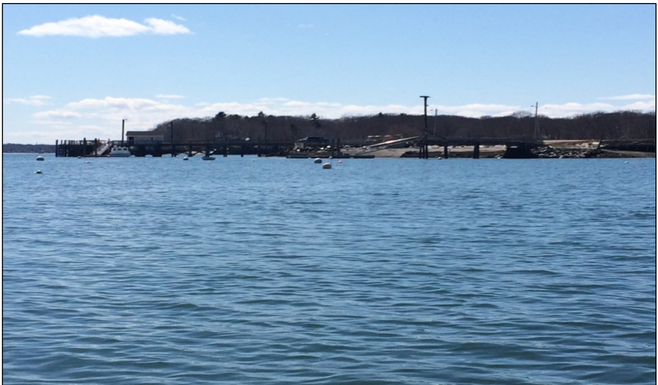
Photograph Two. Facing westerly - view of ferry landing and surrounding development within the vicinity of the project site. Photographer: Tim Forrester, ECO-ANALYSTS, INC. Date: April 13, 2016.
