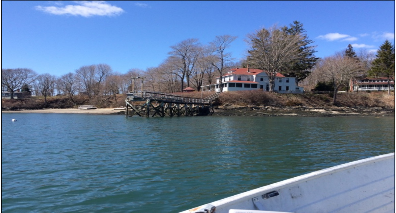
Photograph One. Facing northwesterly from coastal wetland - View of existing pier portion of dock and surrounding development. Photographer: Tim Forrester, ECO-ANALYSTS, INC. Date: April 13, 2016.
