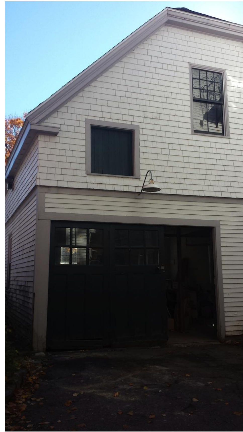
PHOTO OF EXISTING GARAGE
