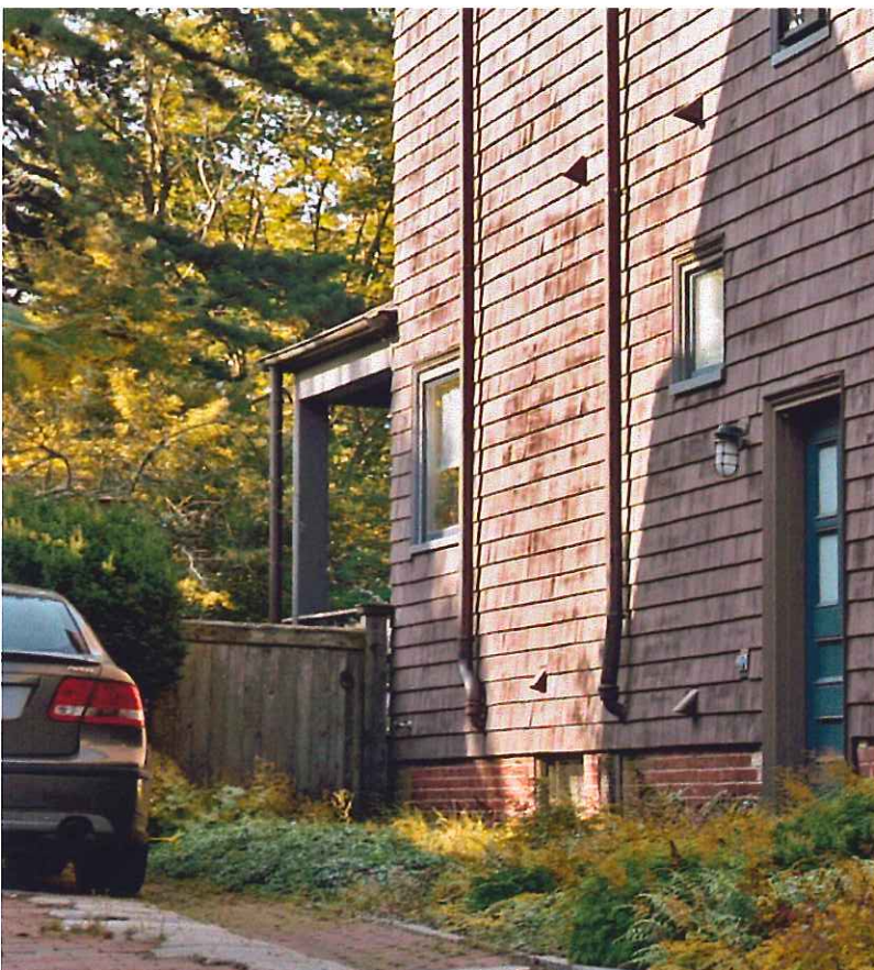
1b Close up; existing window detail
