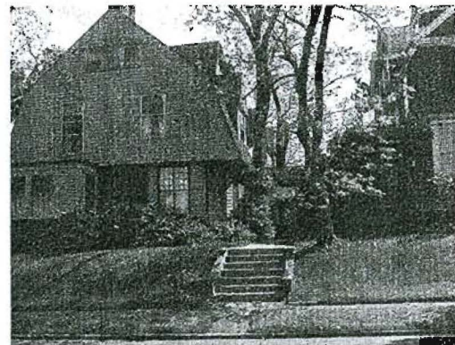
View From Bowdoin Street
