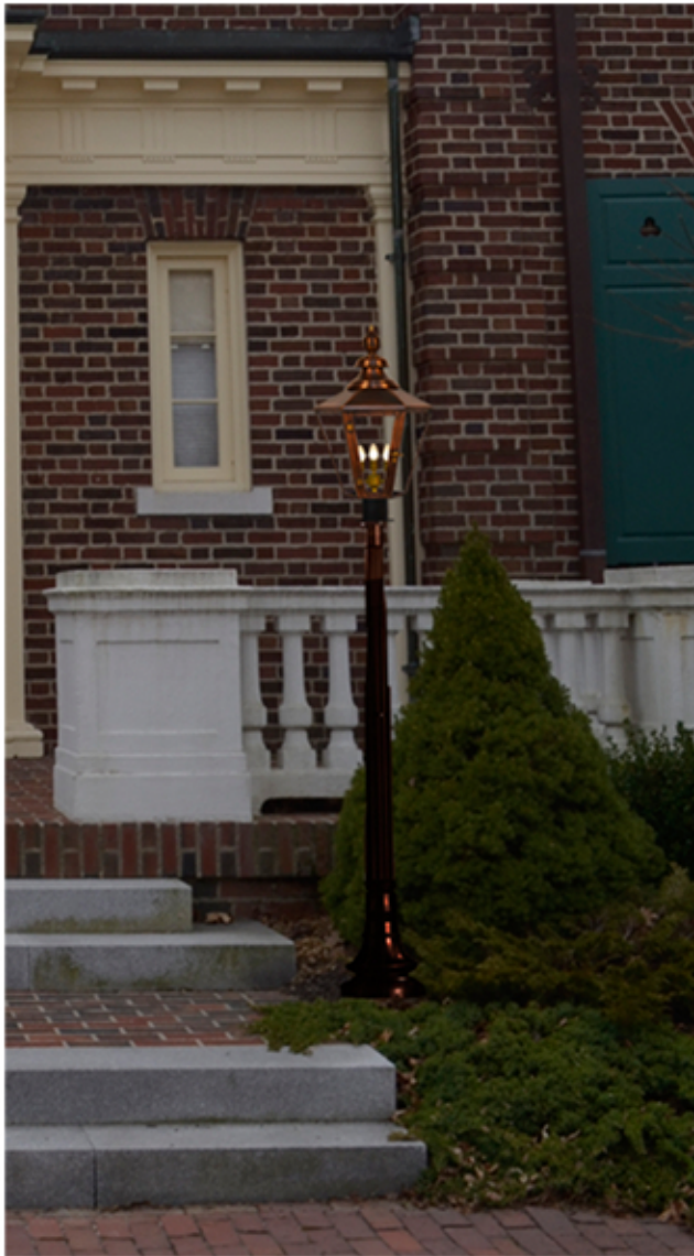
Gas Lamp @ Garage & Front Entry
