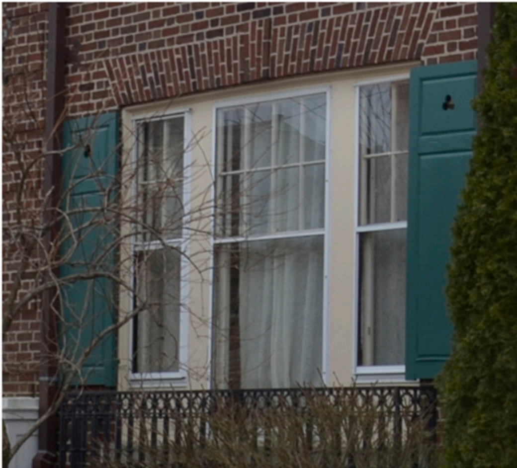
Typical Existing Exterior Storm Window
