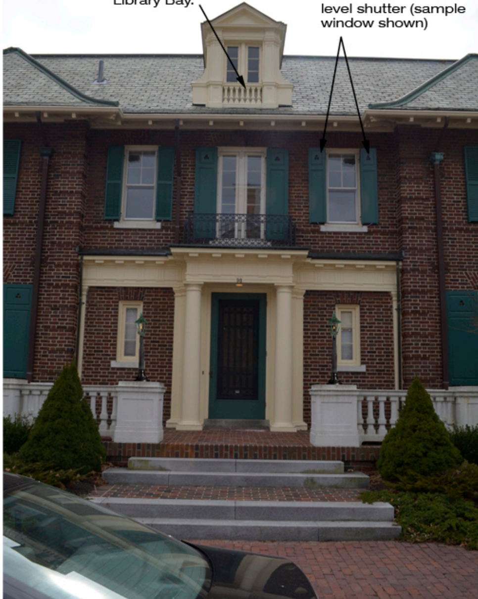
North View - Front Entrance
