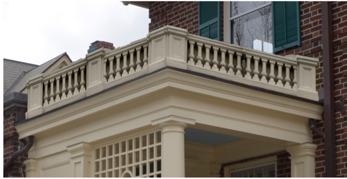
Railing with Back Panel Behind Balusters
