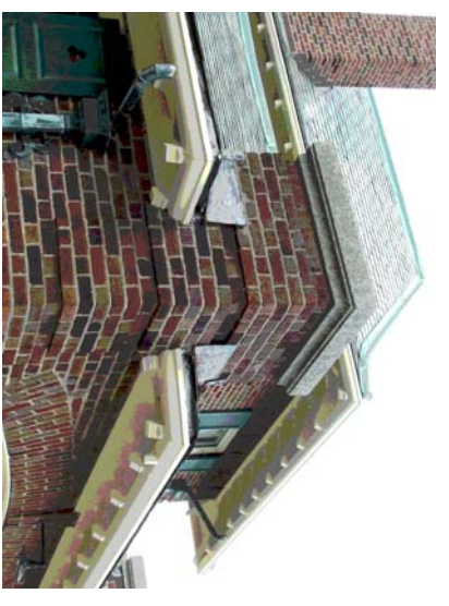
damaged brick at stair treads
