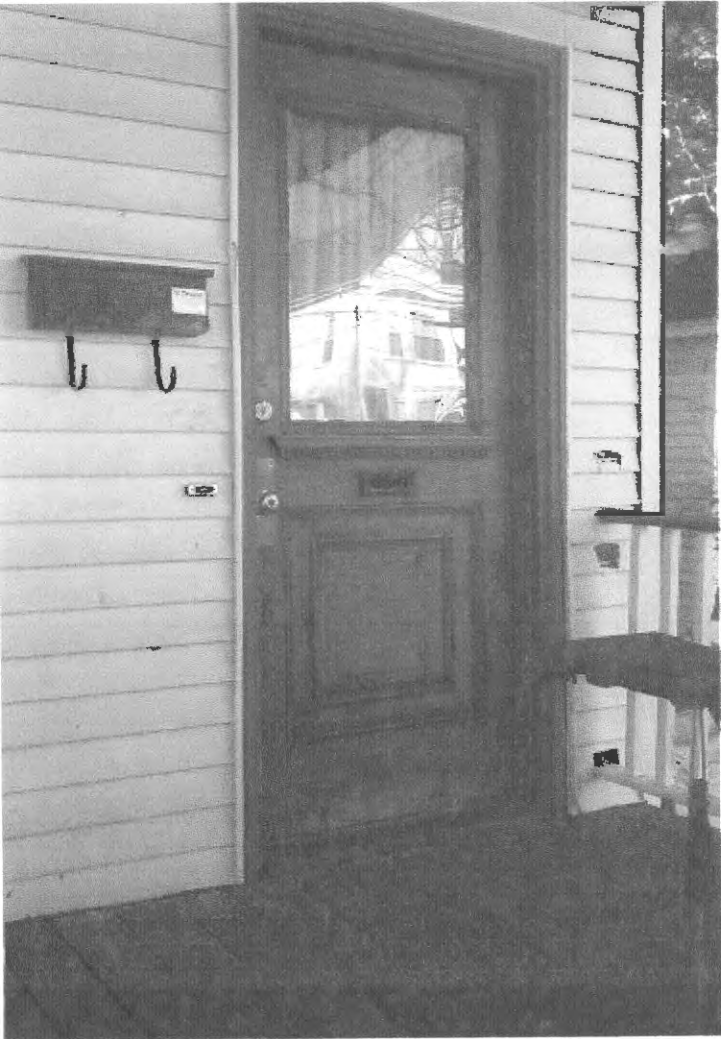
Front Door Right Entrance
