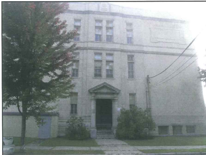
PHOTO 1 – Payson Street Entrance
