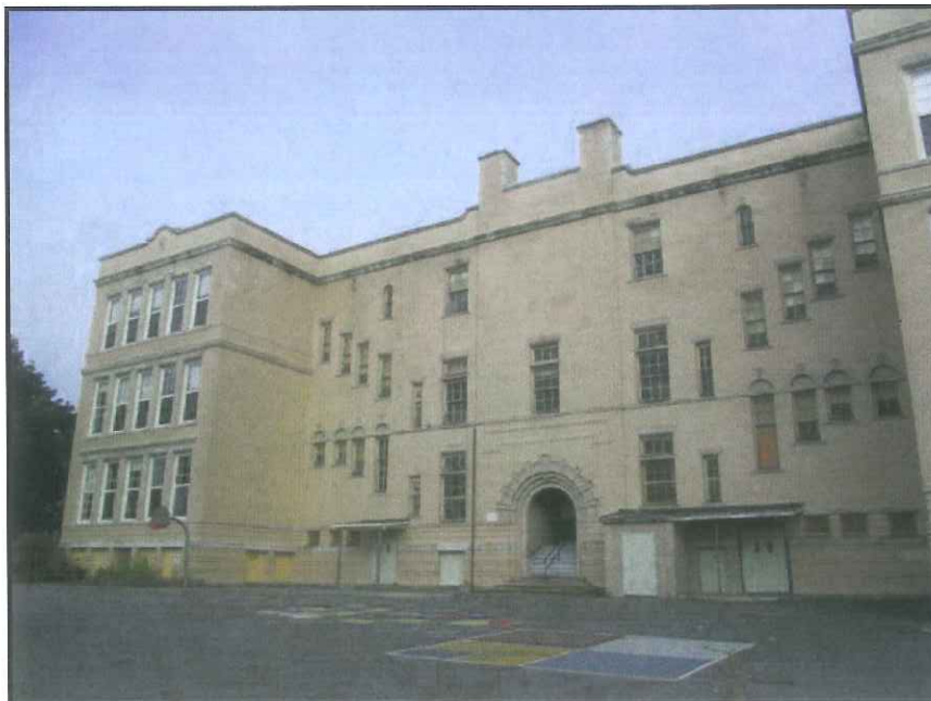
PHOTO 3 – Rear of Building
