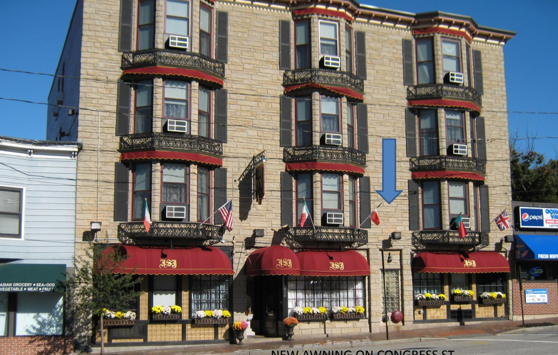
NEW AWNING ON CONGRESS ST FRONTAGE
