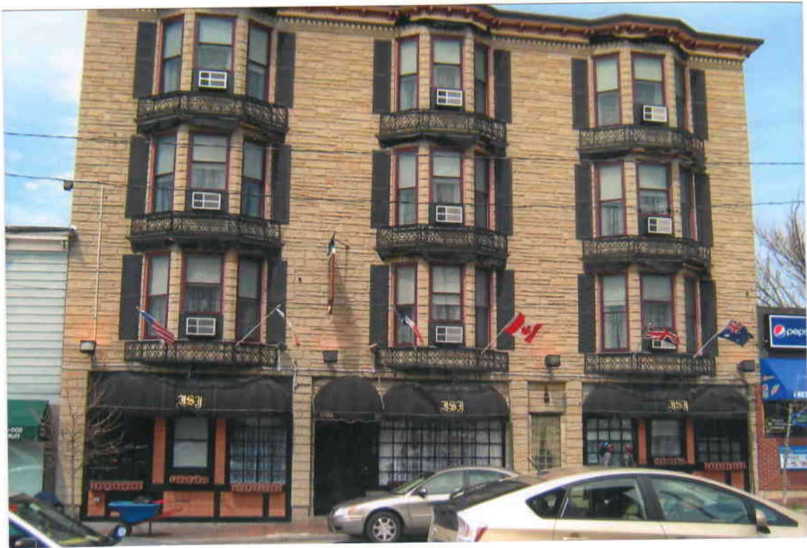
Photo of existing facade awnings
