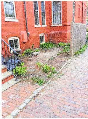
View of existing Patio
