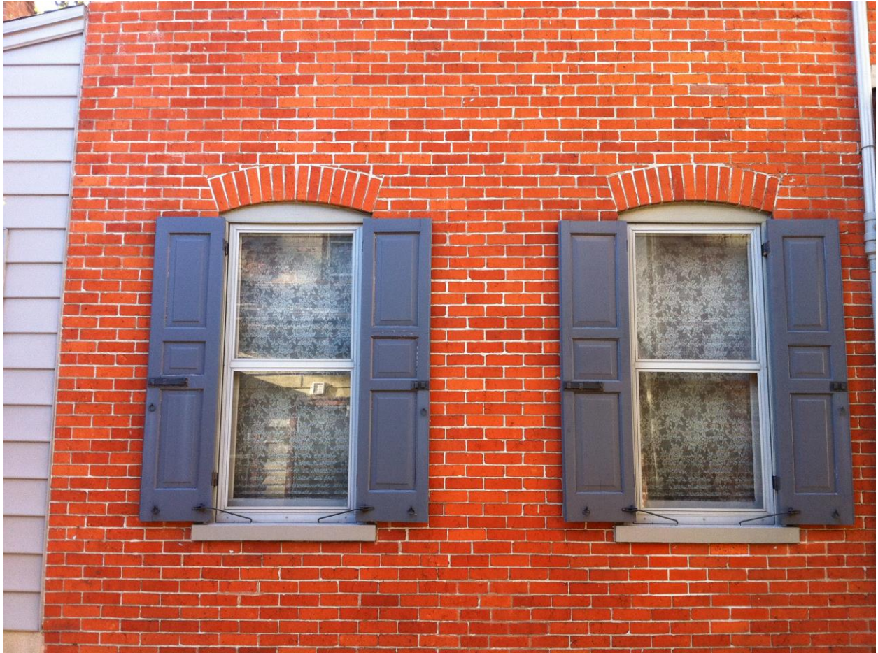
Example of Allied storm windows installed Model HOL-C Window size: approximately 66" x 30"
