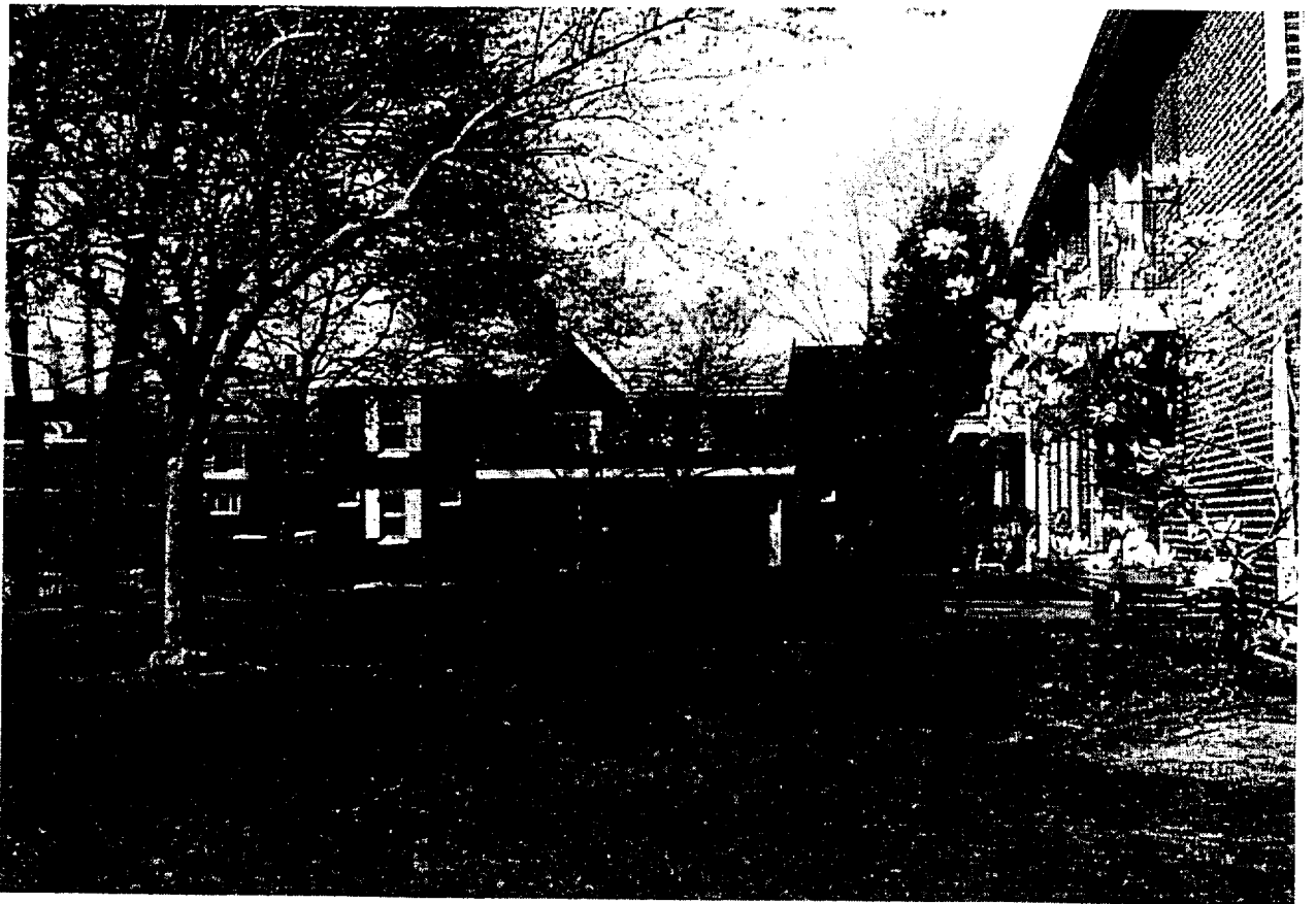
4. View of south façade from Pine Street.
