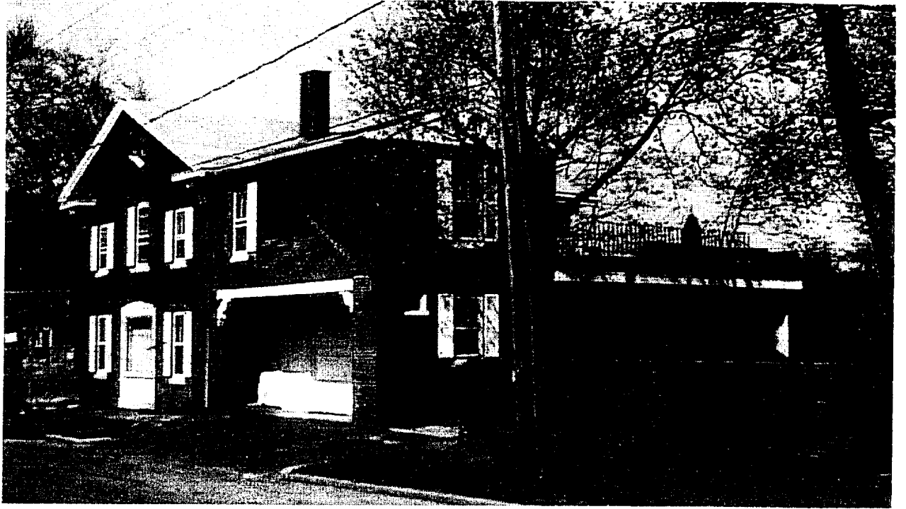
3. View of west and south facades.
