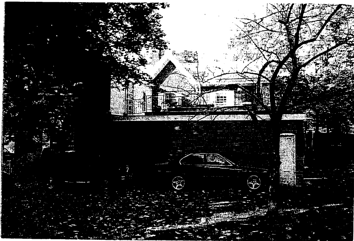
8. VIEW OF SOUTH FACADE
