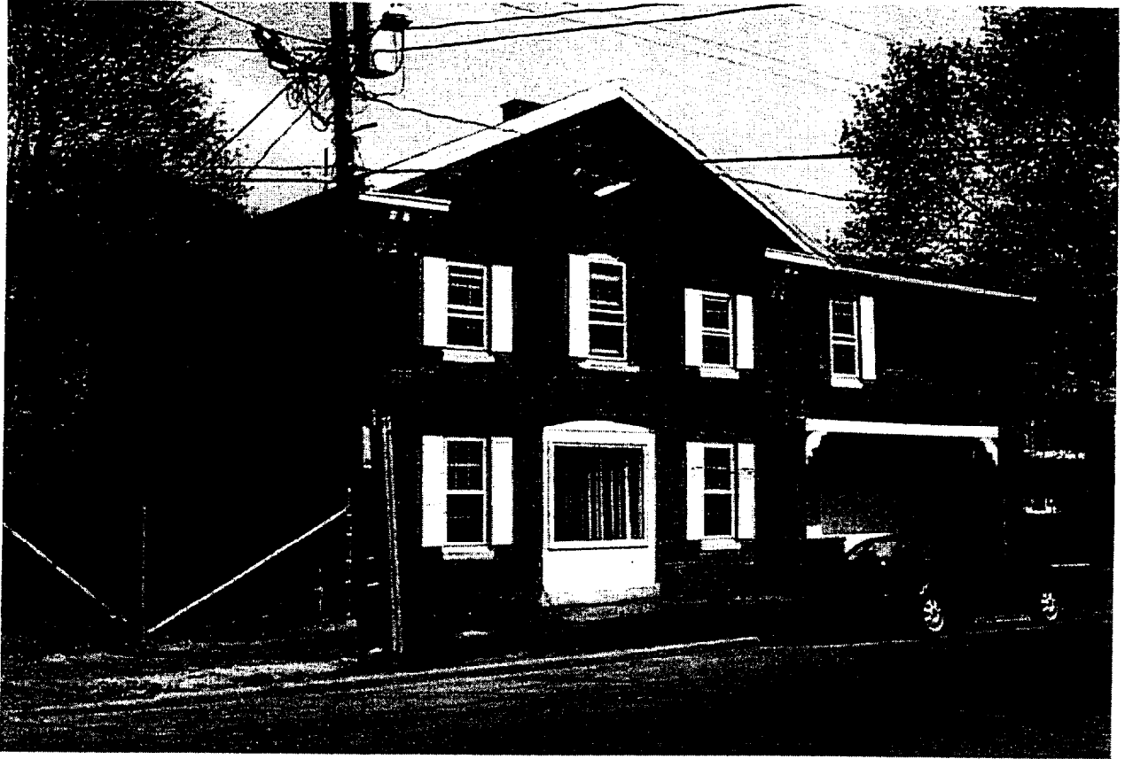
1. View of north and west facades.
