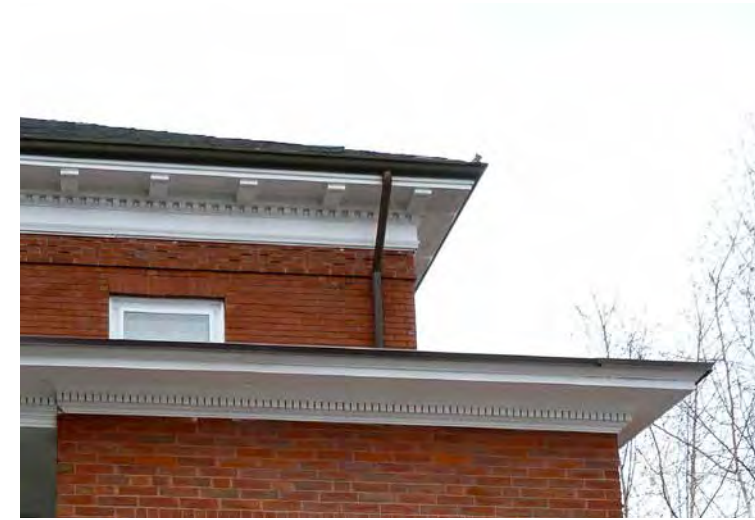
104 West Street. Detail of existing rear porch cornice.
