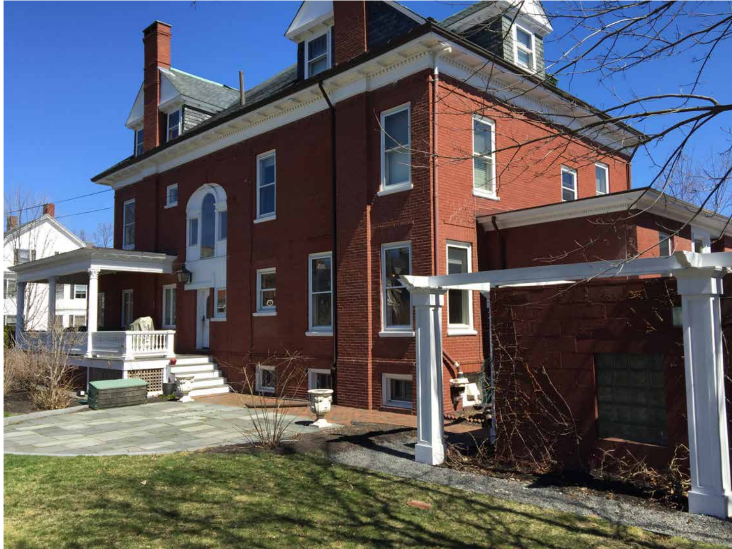
104 West Street. View from southwest corner showing west (garden) facade.
