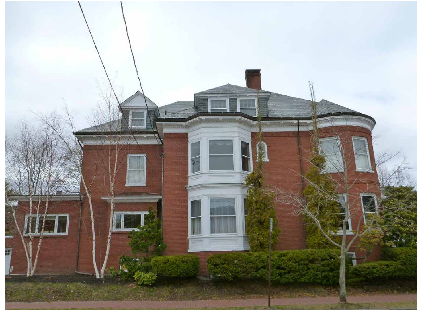
104 West Street. Chadwick Street facade.
