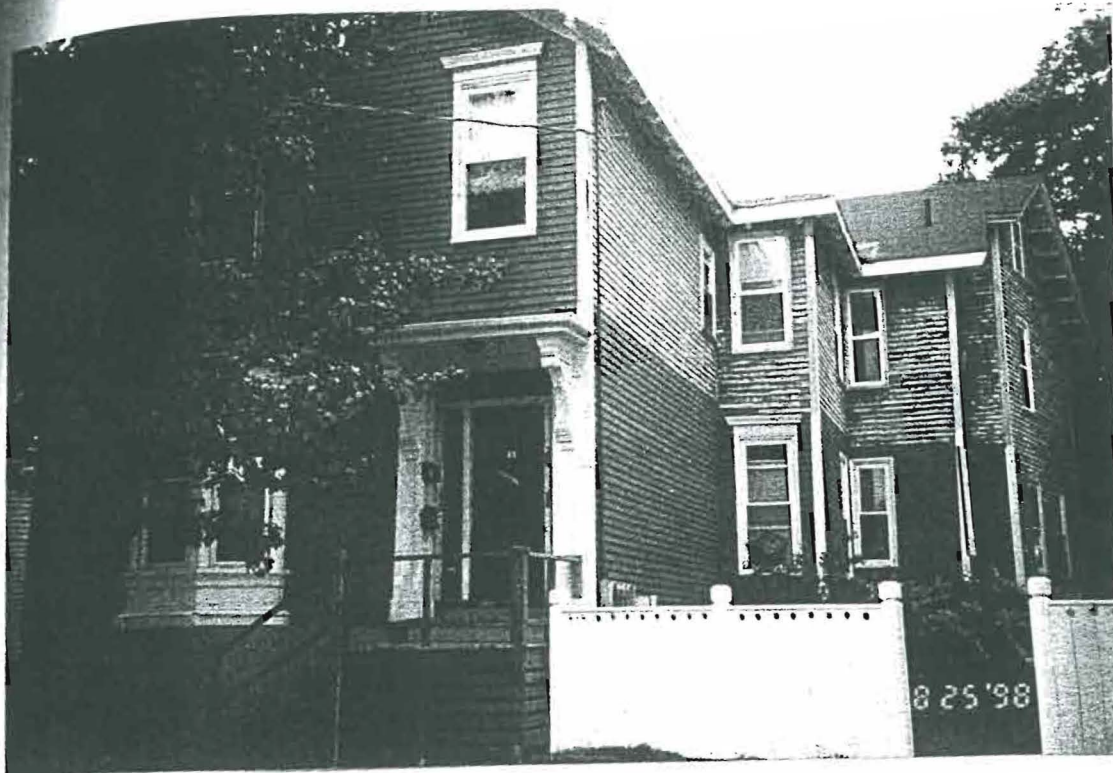
CARLETON STREET APARTMENTS.
