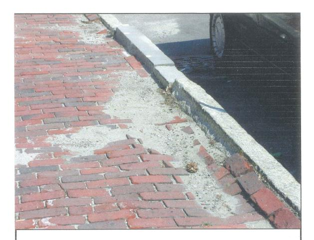
Above: Sidewalk damage along the granite curbing Below: Damage at the existing staircase and wall
