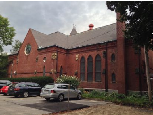
West facade facing parking lot - featuring significant stained glass windows
