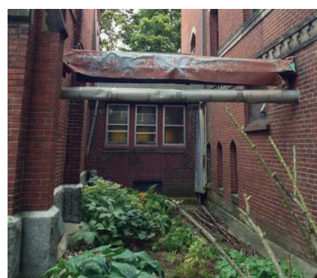
West facade of 'Connector' piece facing parking
