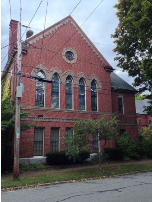
East facade facing Thomas Street
