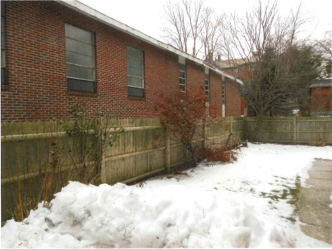
Wood fence along south property line to be removed and replaced with a new 6' solid board fence with a 2' finial topper and decorative caps.
