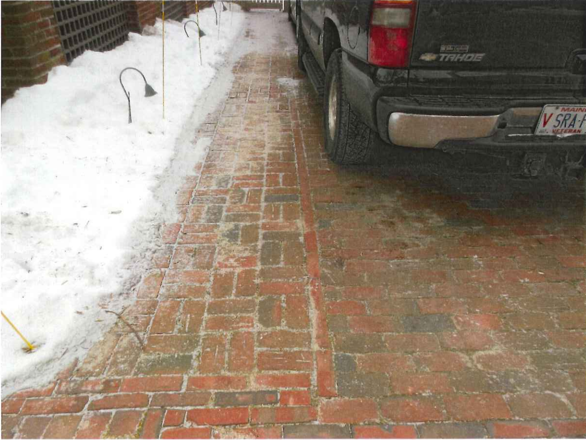
Example of brick and patterns to be used: basket weave for the walkway, running bond for the driveway. This is a picture of the walkway and driveway currently found at 40 Neal Street, Portland.
