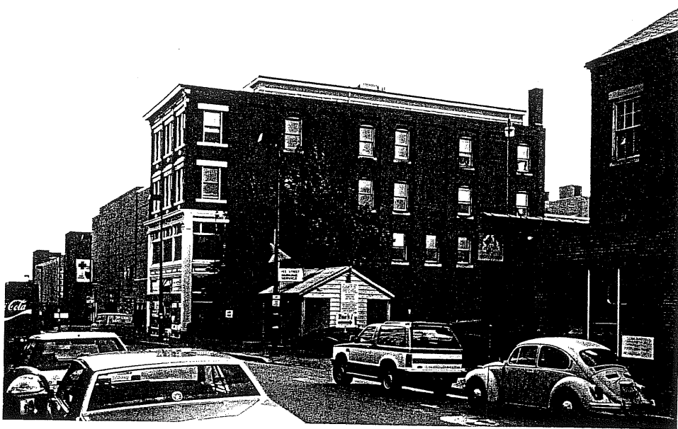
By locating the rooftop addition back from the streetwall, the original architectural integrity of the building is retained.
