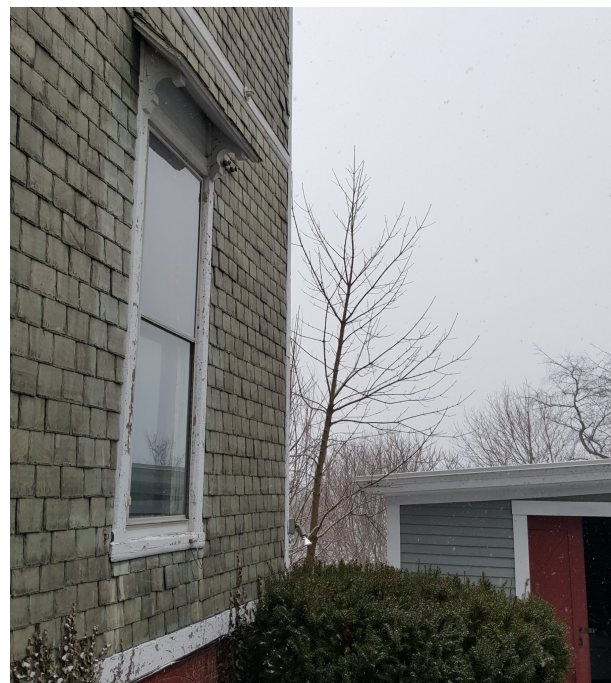
WINDOW TRIM ON HOUSE PHOTO
