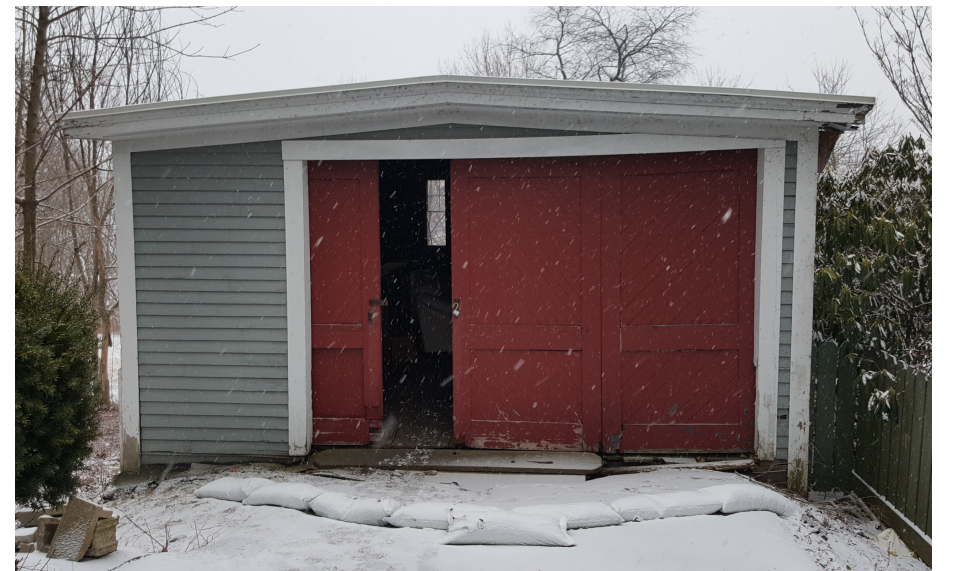
EXISTING GARAGE FRONT/NORTH PHOTO
