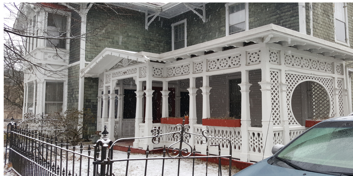
EXISTING HOUSE PORCH PHOTO
