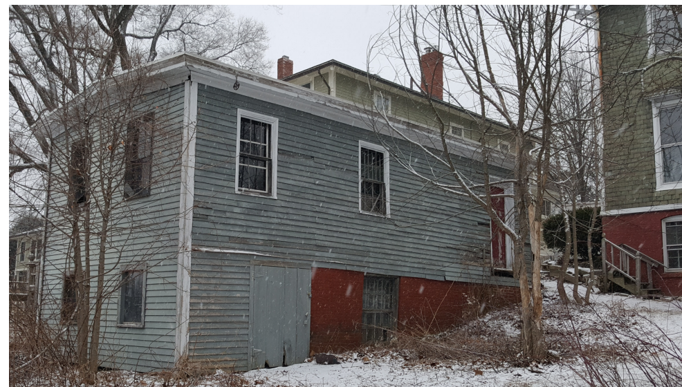
EXISTING GARAGE SOUTH EAST CORNER PHOTO
