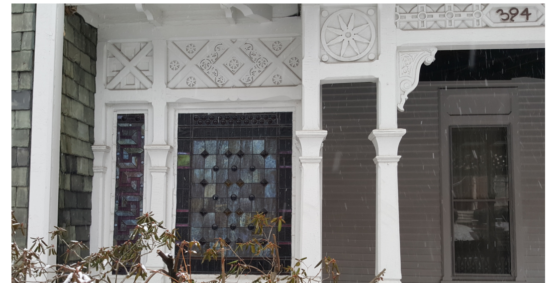
EXISTING ENTRY PHOTO
