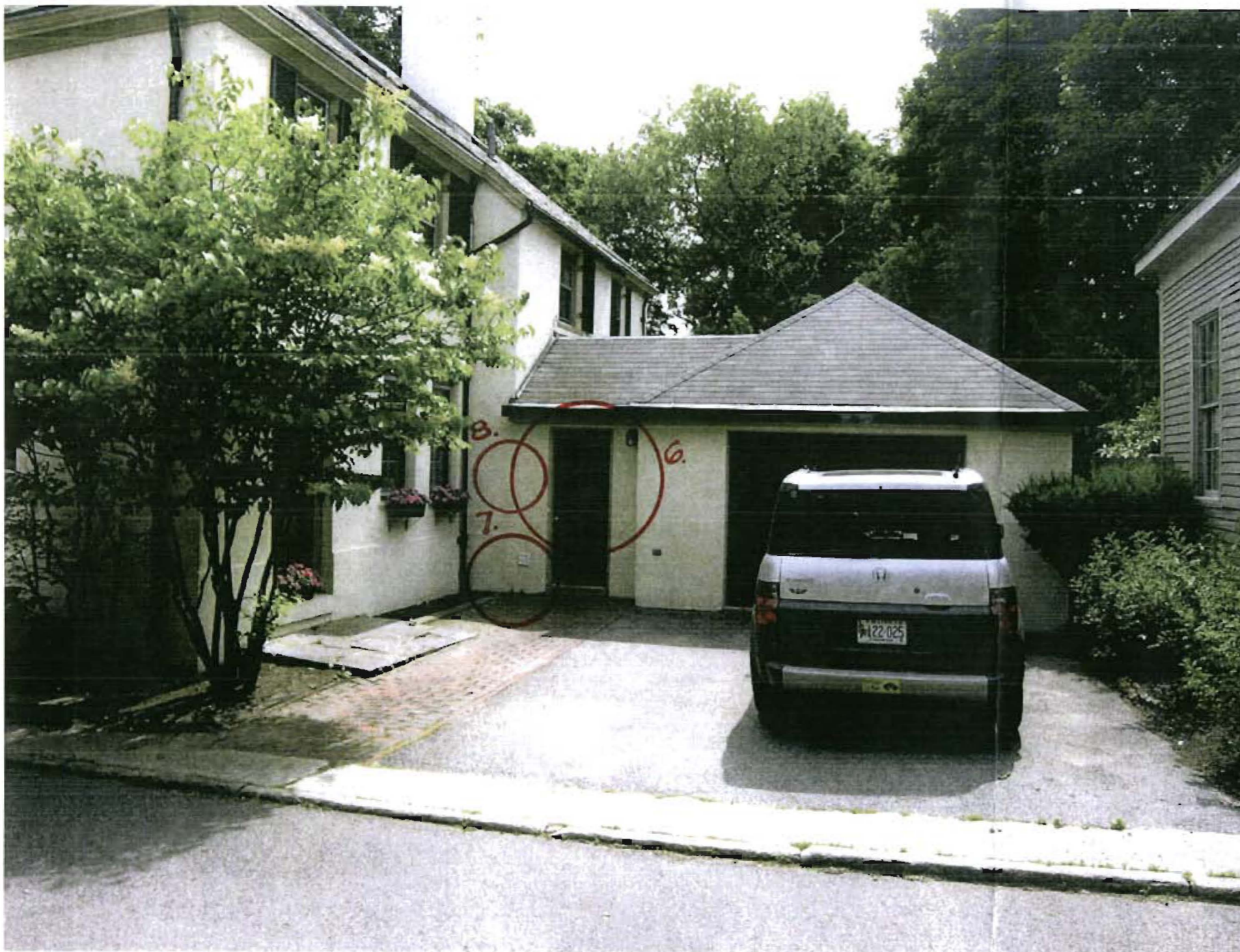
PHOTO VIEW OF EXISTING SIDE (east) ELEVATION
