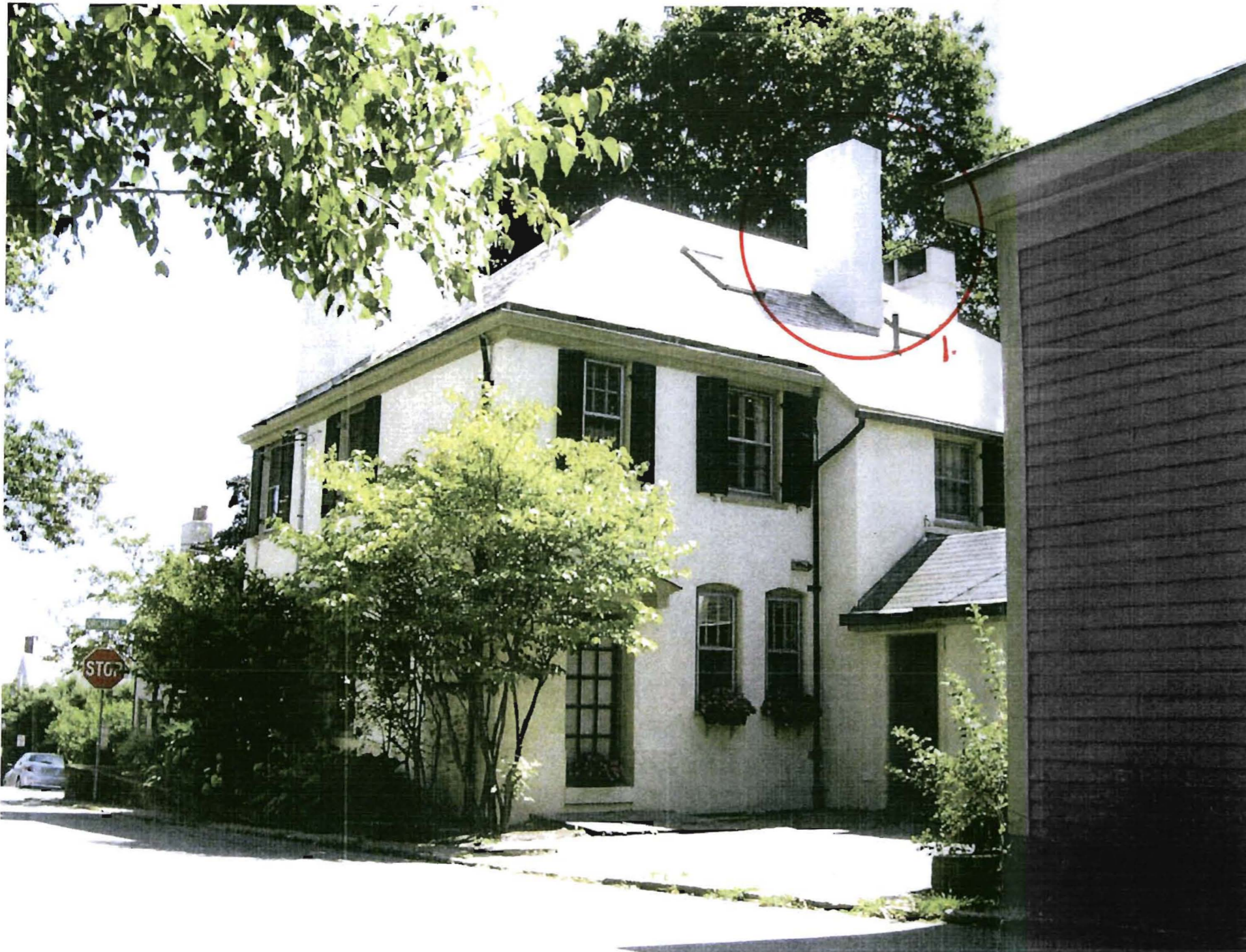
PHOTO VIEW OF EXISTING REAR (north) ELEVATION
