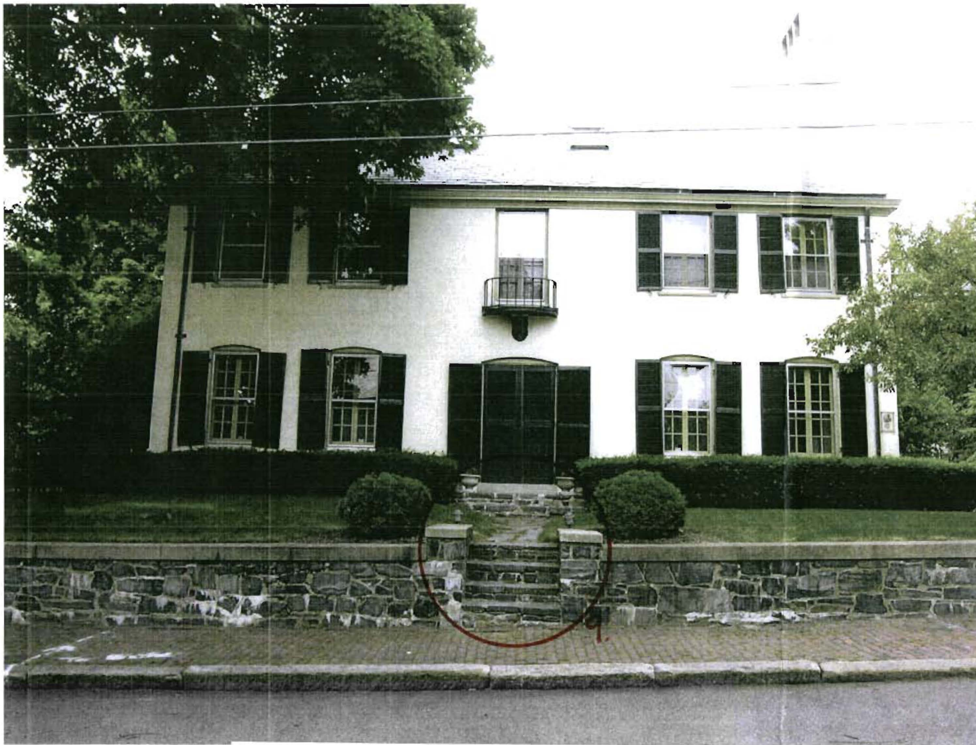
PHOTO VIEW OF EXISTING FRONT (south) ELEVATION
