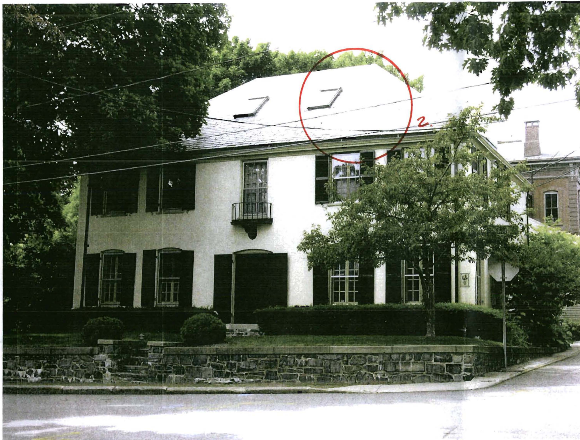
PHOTO VIEW OF EXISTING FRONT (south) ELEVATION
