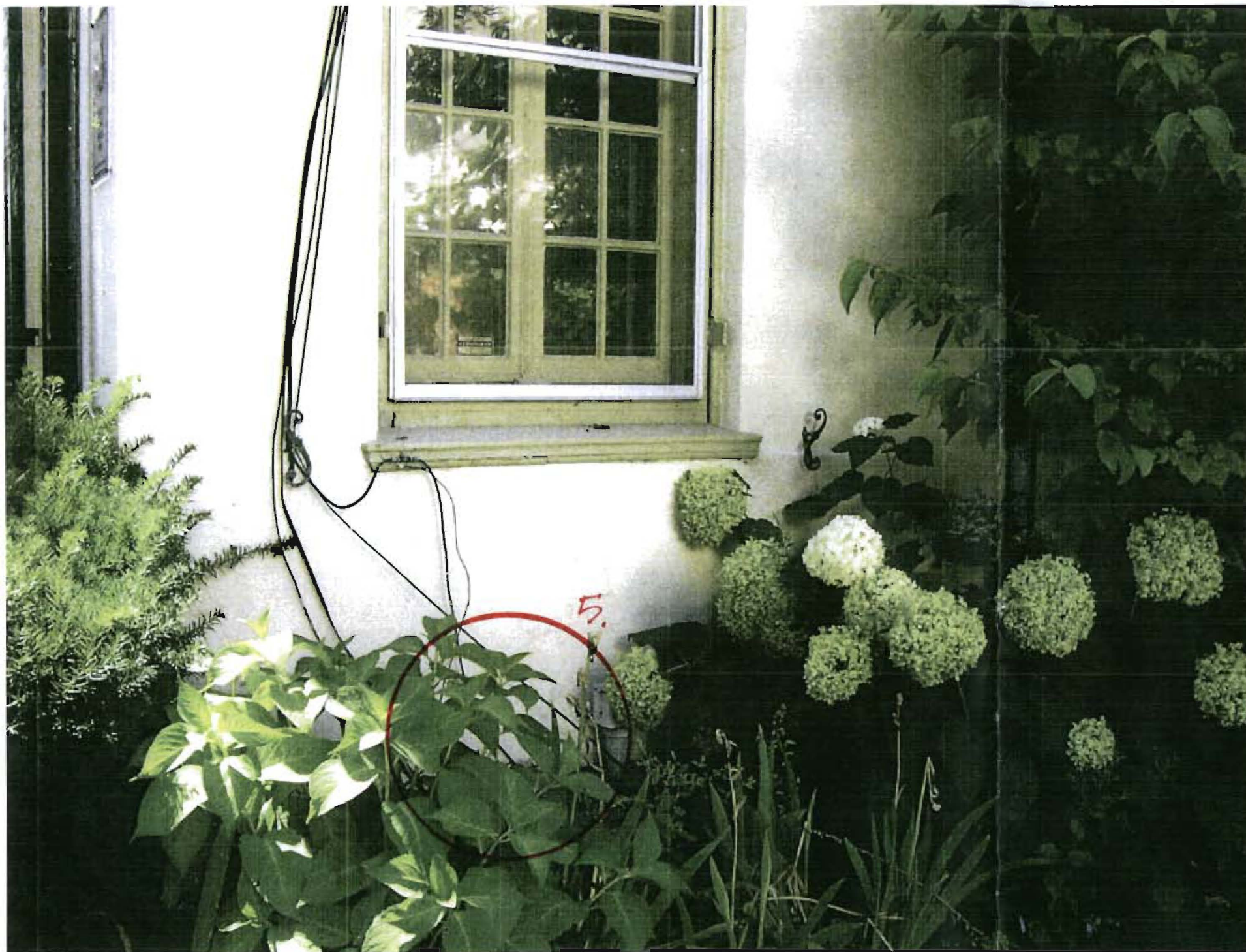
PHOTO VIEW OF EXISTING SIDE (east) ELEVATION
