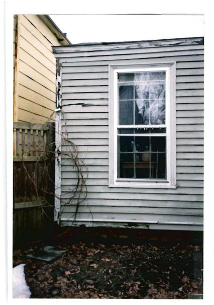
as you can see the lack of 6 overhang on the back section is architecturally inconsistent with the front and encourages delectionation due to rot.
