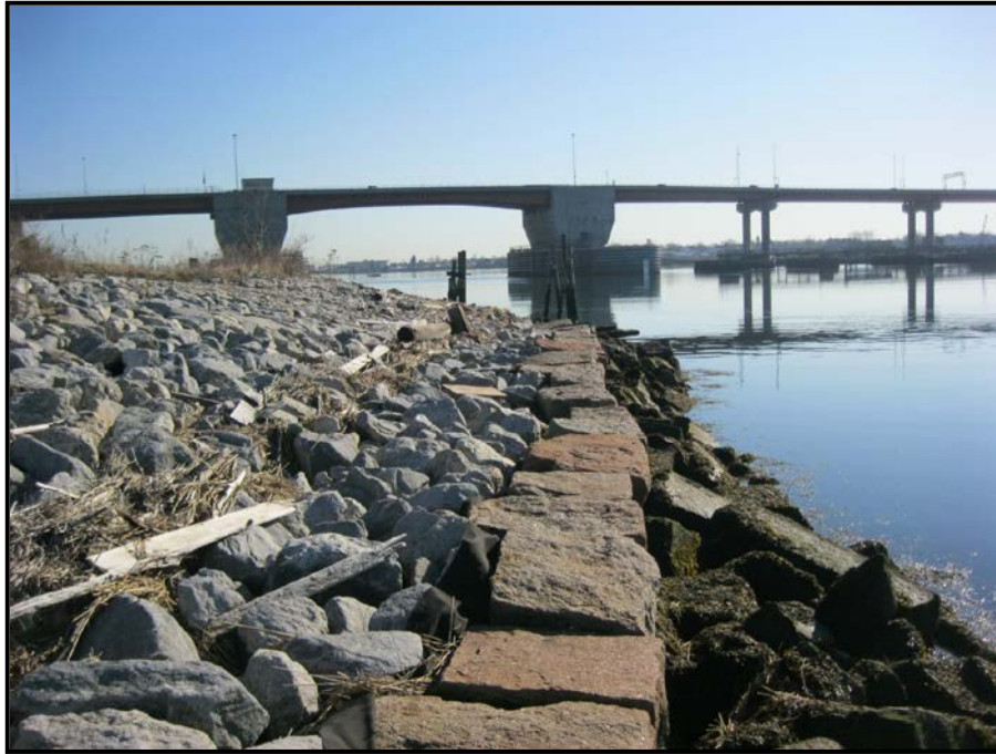
PHOTO 3 – Existing Granite Revetment
