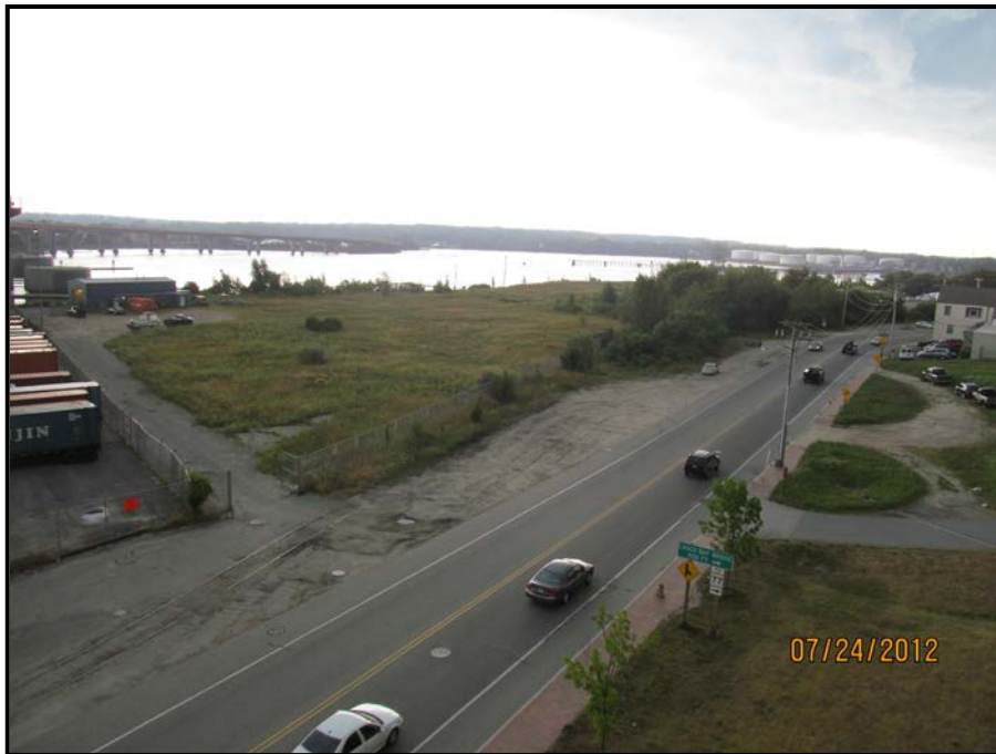
PHOTO 2 – View from Bridge Onramp
