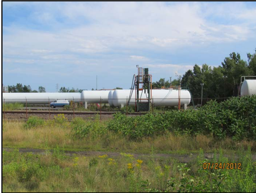
PHOTO 3 – Existing Gas Tanks
