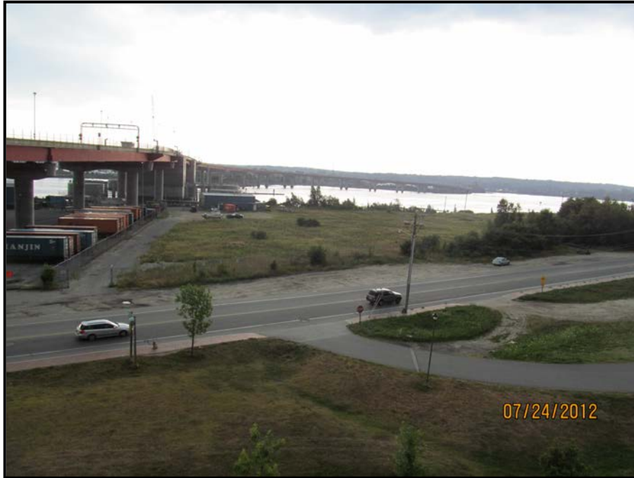
PHOTO 1 – View from the North
