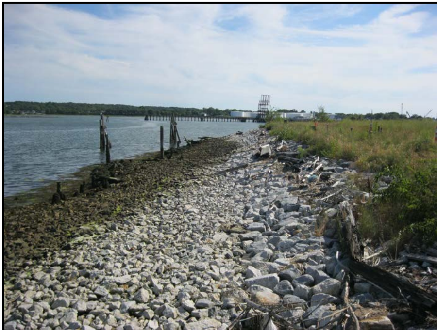
PHOTO 4 – Riprap Stabilized Shorefront – Unutil Parcel
