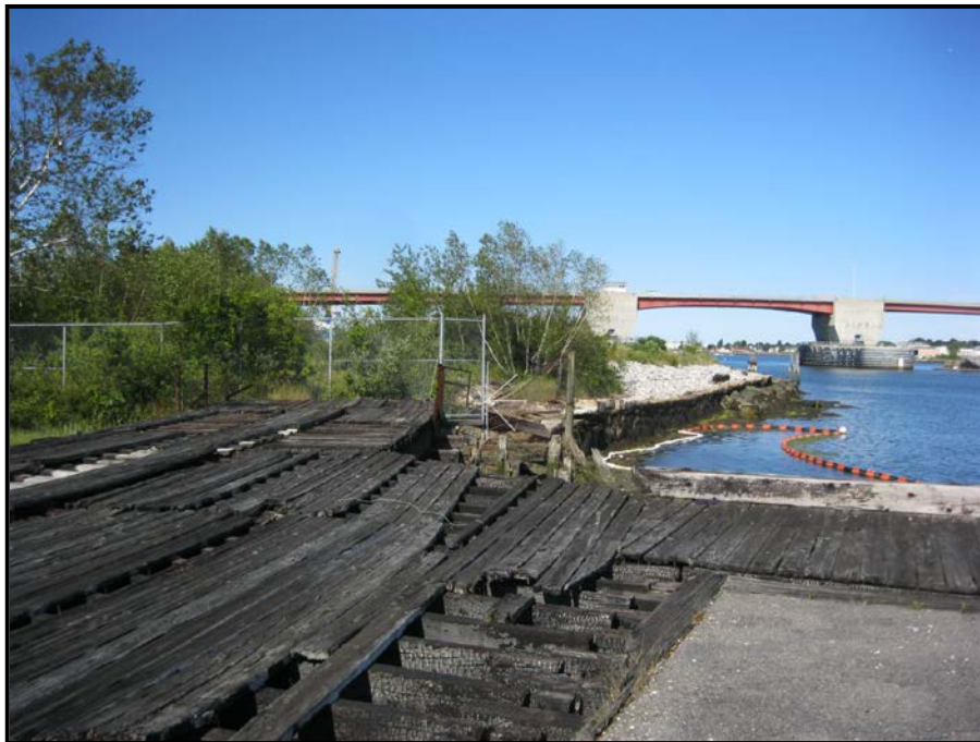
PHOTO 2 – Easterly End Pier
