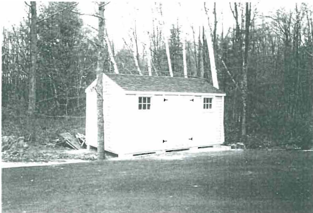
Note: Typical wood frame/asphalt shingle shed building.
