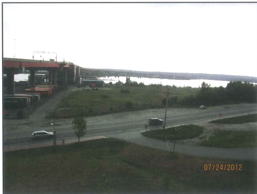
PHOTO 1 – View from the North
