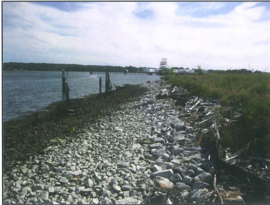
PHOTO 4 – Riprap Stabilized Shorefront – Unutil Parcel
