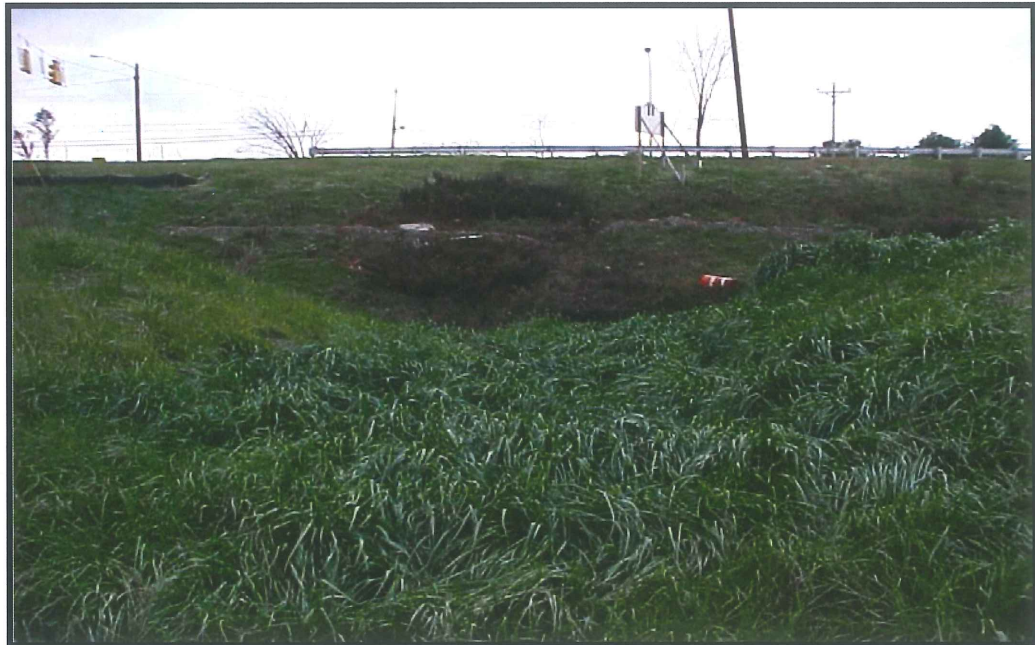
A WELL STABILIZED VEGETATED SWALE SHOWS LITTLE SIGNS OF EROSIVE VELOCITIES OR FLOWS. THIS SWALE ALSO FUNCTIONS AS A POND SPILLWAY
