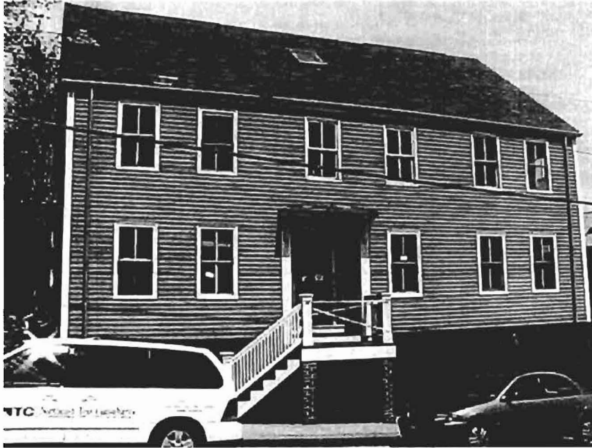
View of front of structure assessed during this event.
